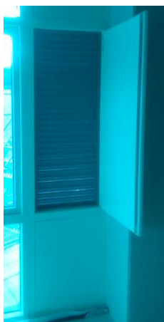
Figure 7.3.3: Example of Acoustic Ventilation Panel (TEK Ltd)
