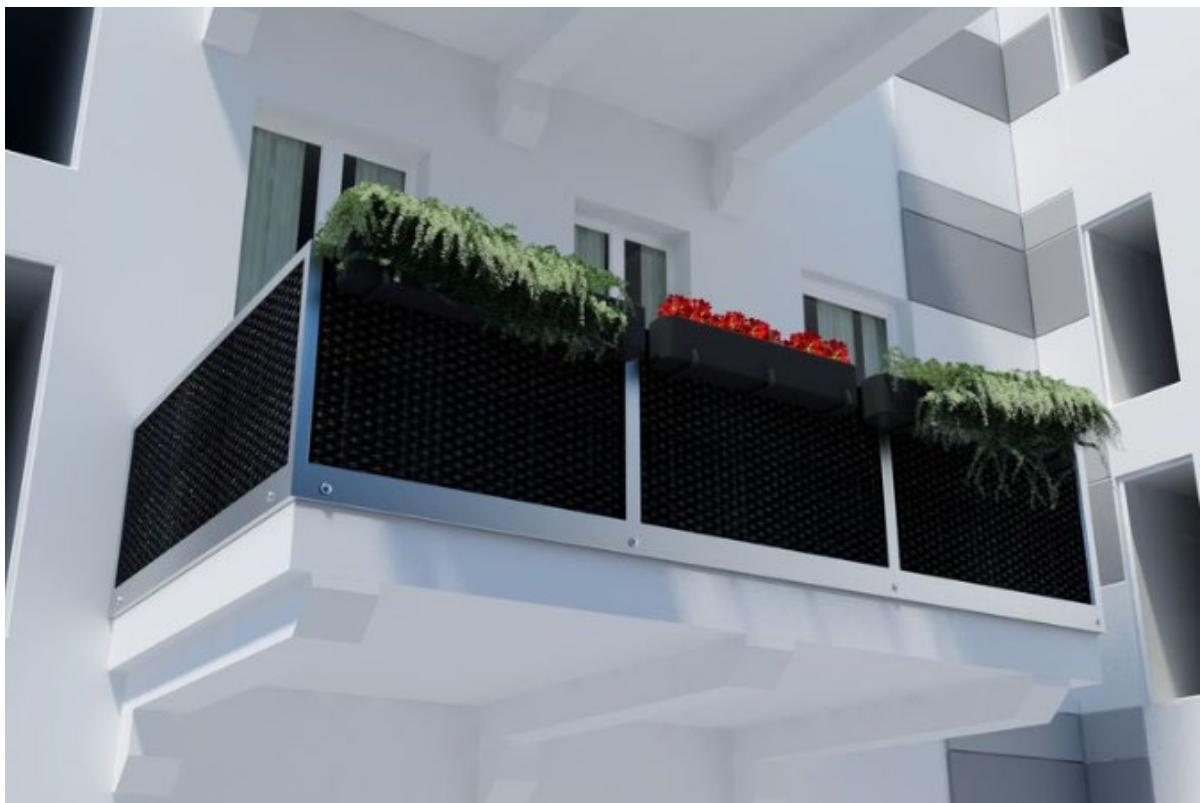
Figure 18 - 50% porous balustrade on balcony
