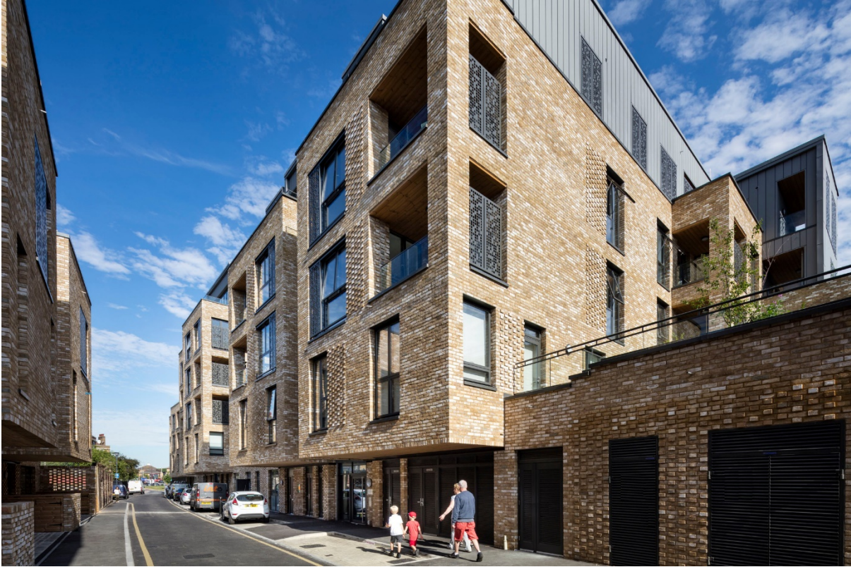
Figure 16 - Porous full height screen on one side of balcony to mitigate corner balconies
