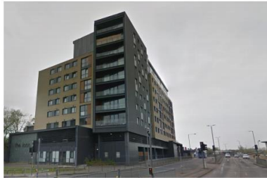
View looking towards site from the Icon
