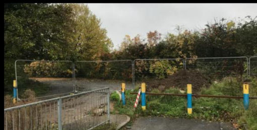
Former entrance to car park
