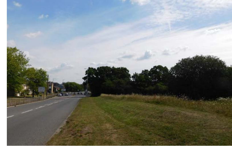
2 Looking East along Laindon Link
