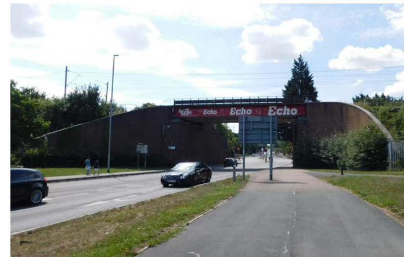
3 Railway bridge adjacent to the site
