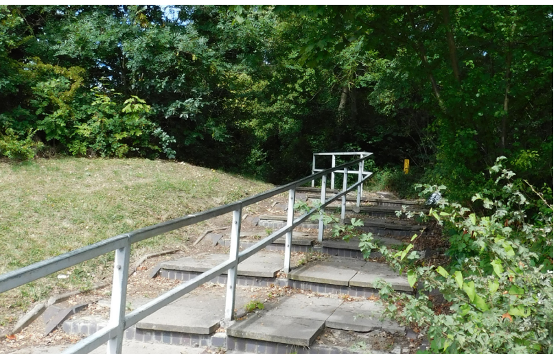
5 Pedestrian link to roundabout underpass
