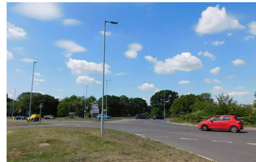
5 View toward the site from opposing roundabout corner
