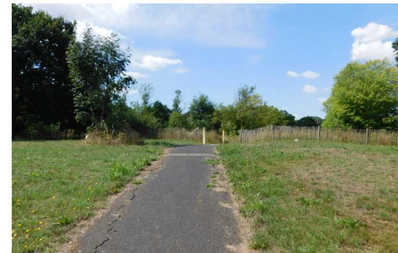
6 Existing pedestrian access
