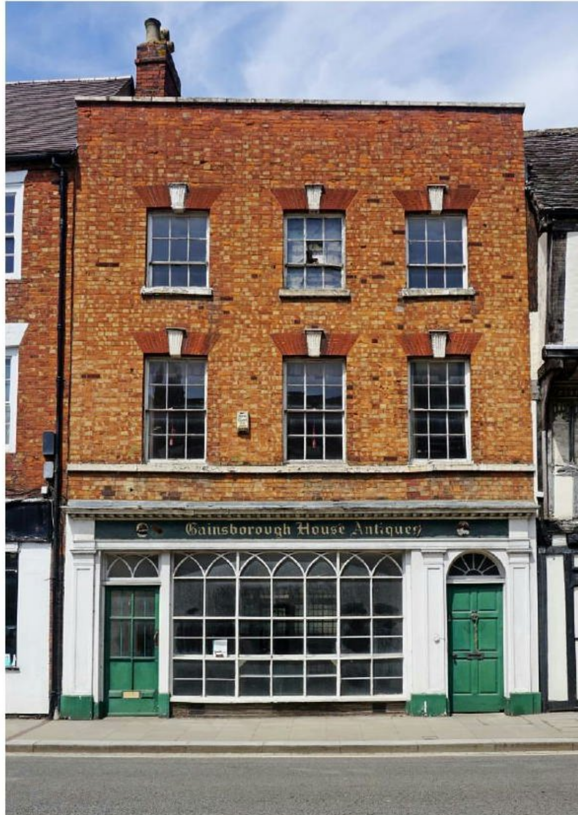
No. 81 Church Street
