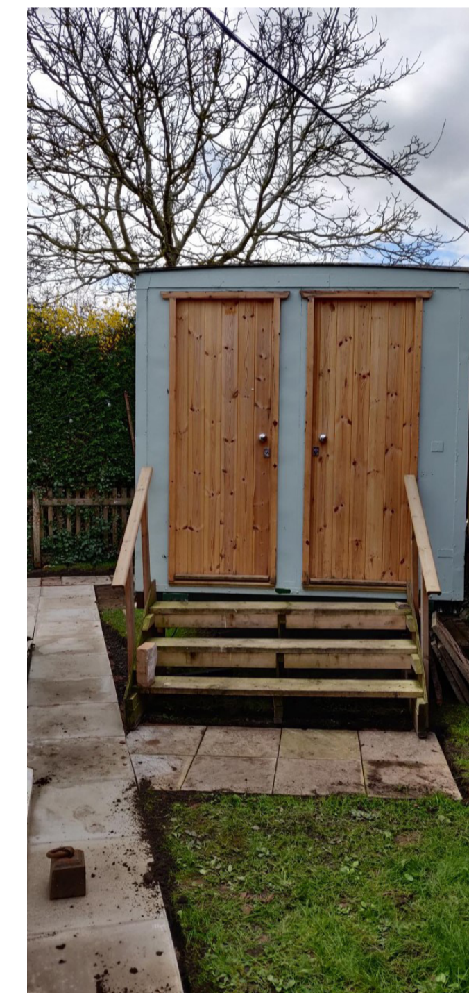
Photo of Toilet Block on site West Elevation
