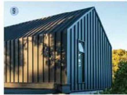
Metal standing facade and roof
