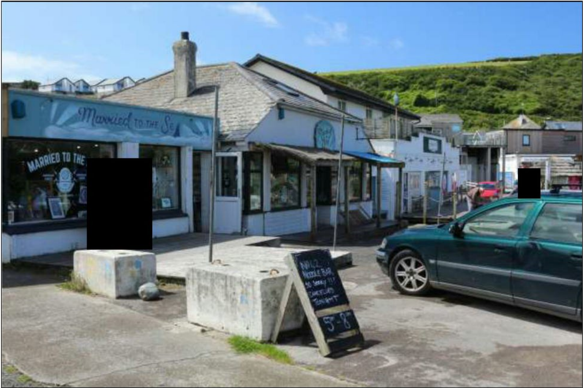
9. BUILDINGS 3-2, VIEWED FROM THE NORTH.
