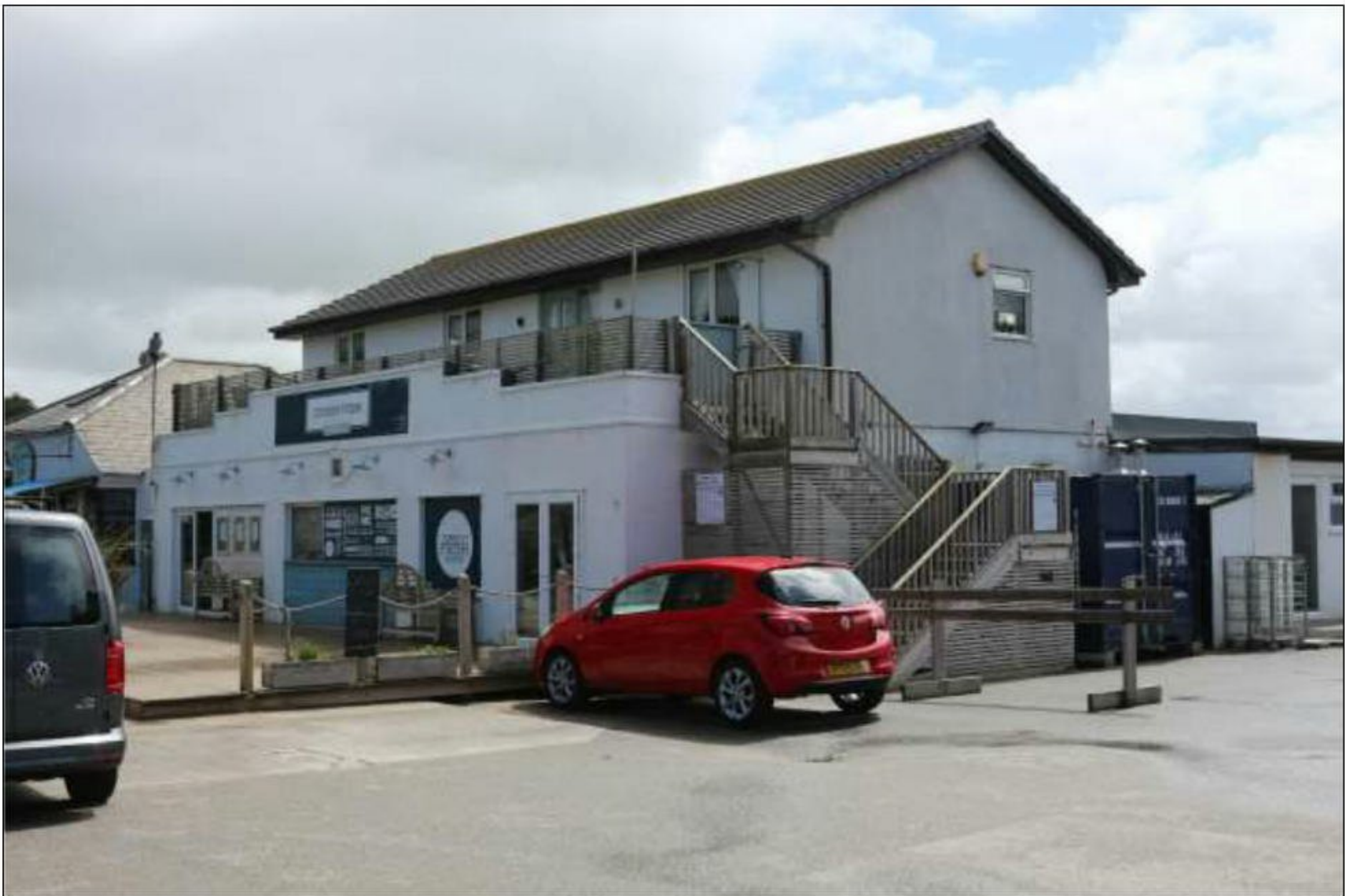
15. BUILDING 1, VIEWED FROM THE WEST.
