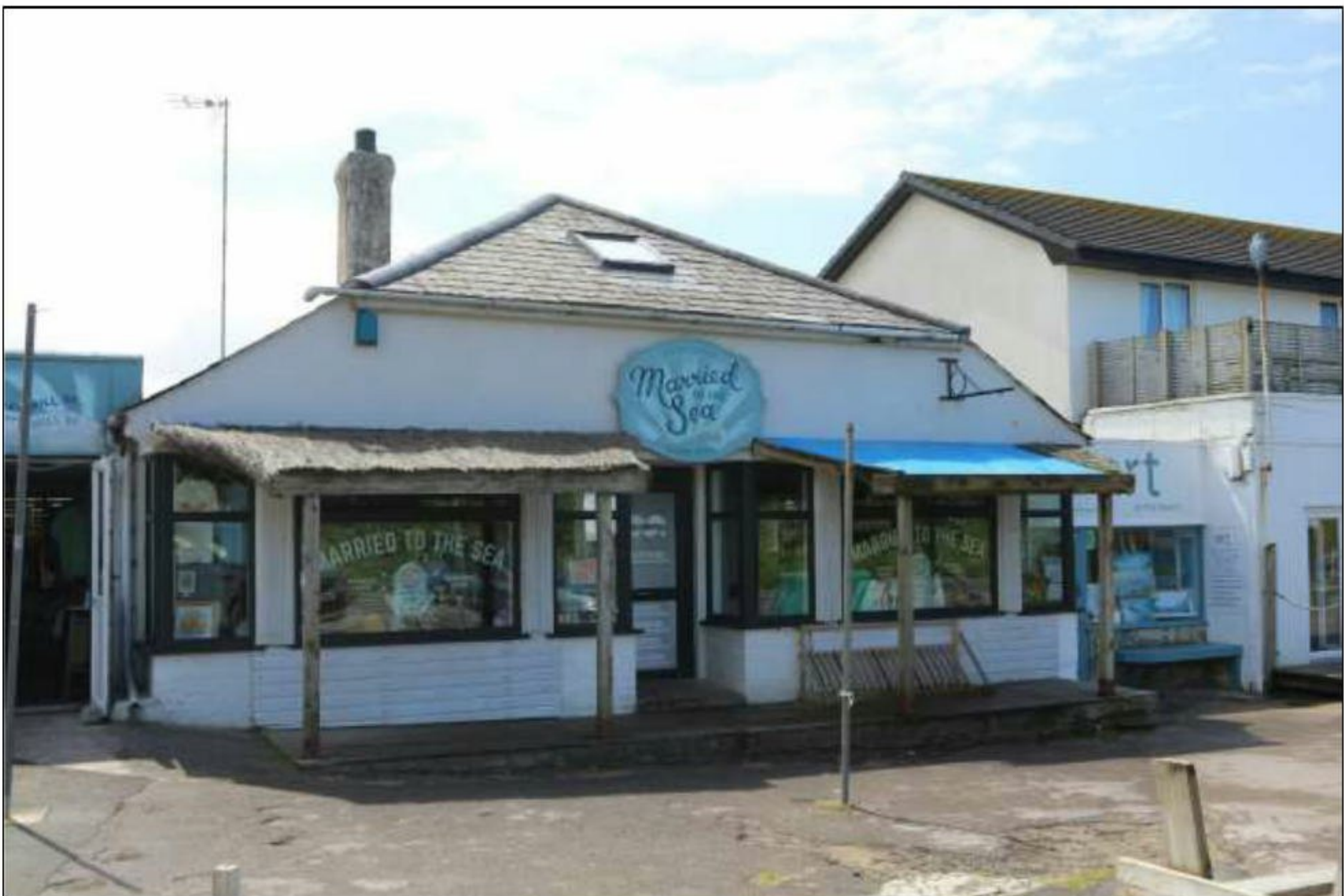
10. BUILDING 2, VIEWED FROM THE WEST.
