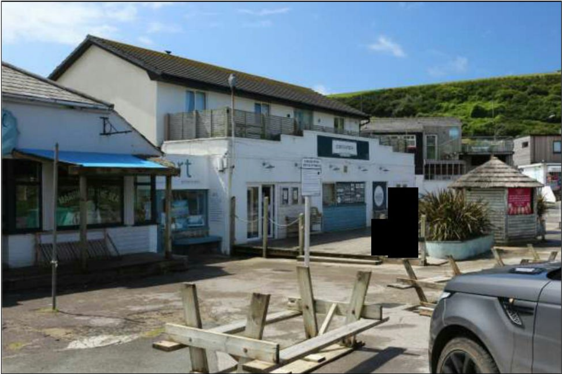
11. BUILDING 1, VIEWED FROM THE NORTH.
