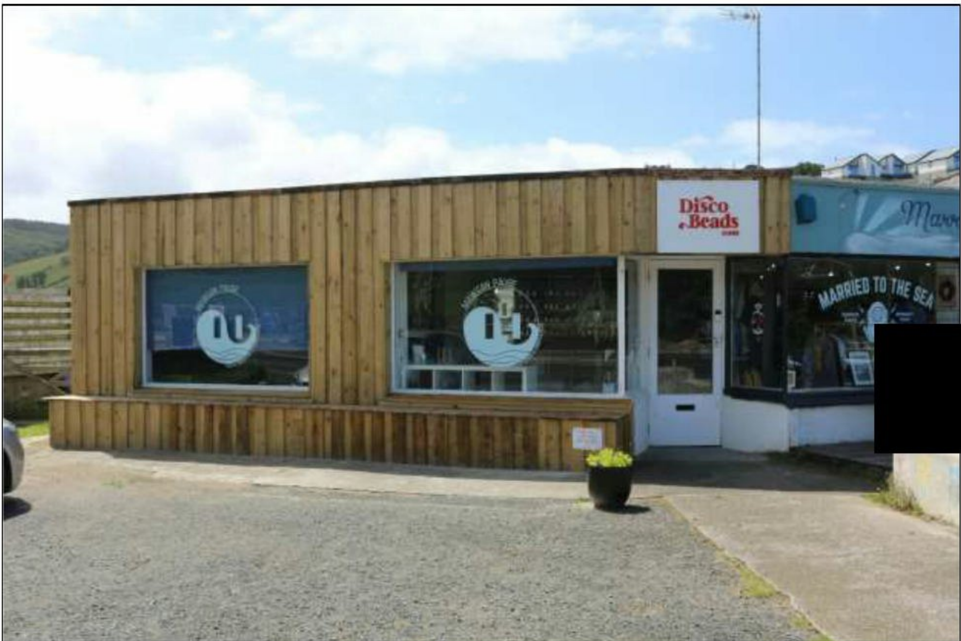
8. BUILDING 3, FROM THE NORTH.
