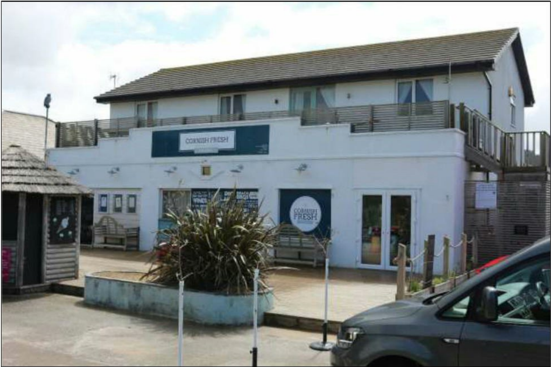
14. BUILDING 1, VIEWED FROM THE WEST.
