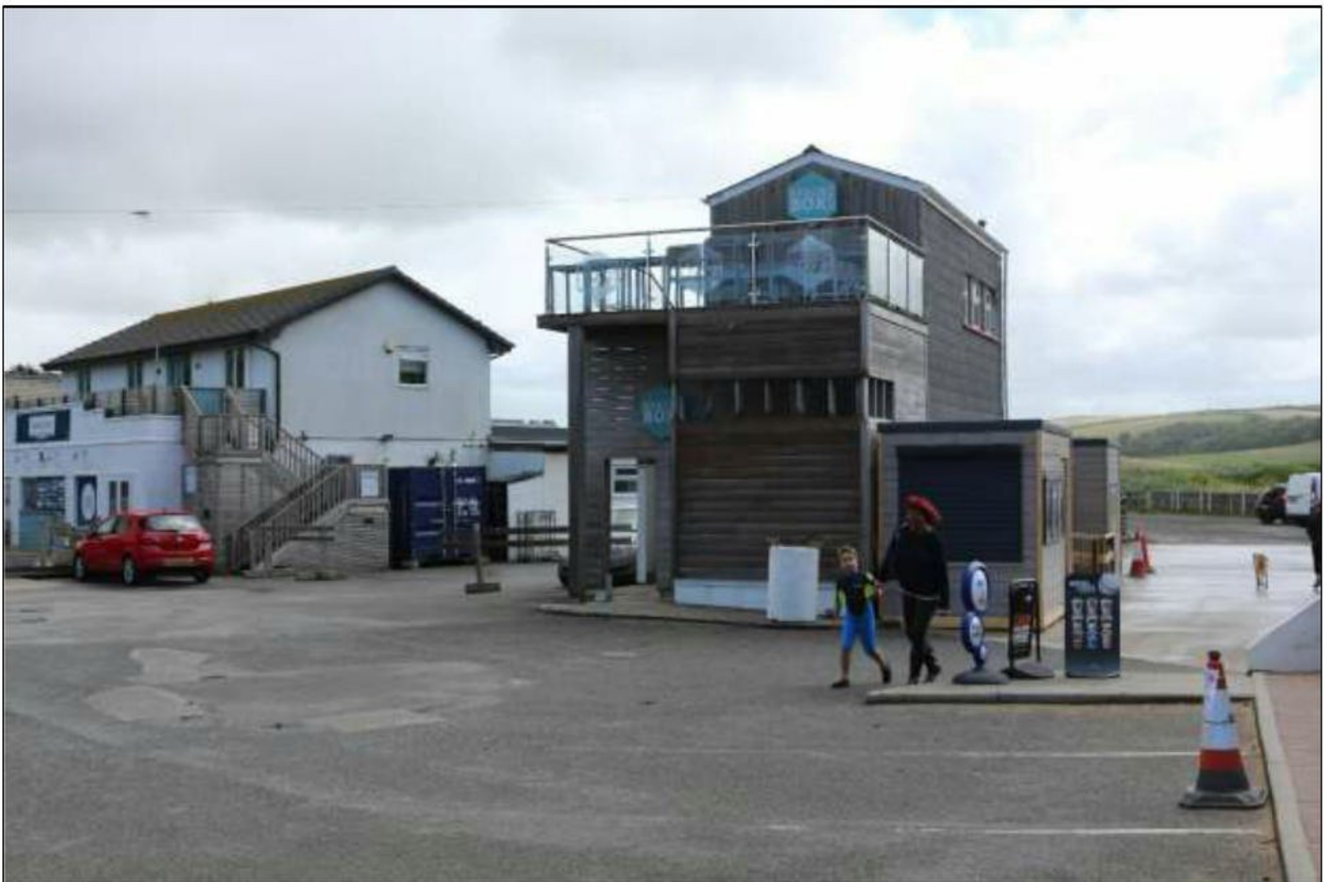
17. BUILDING 4, VIEWED FROM THE WEST.
