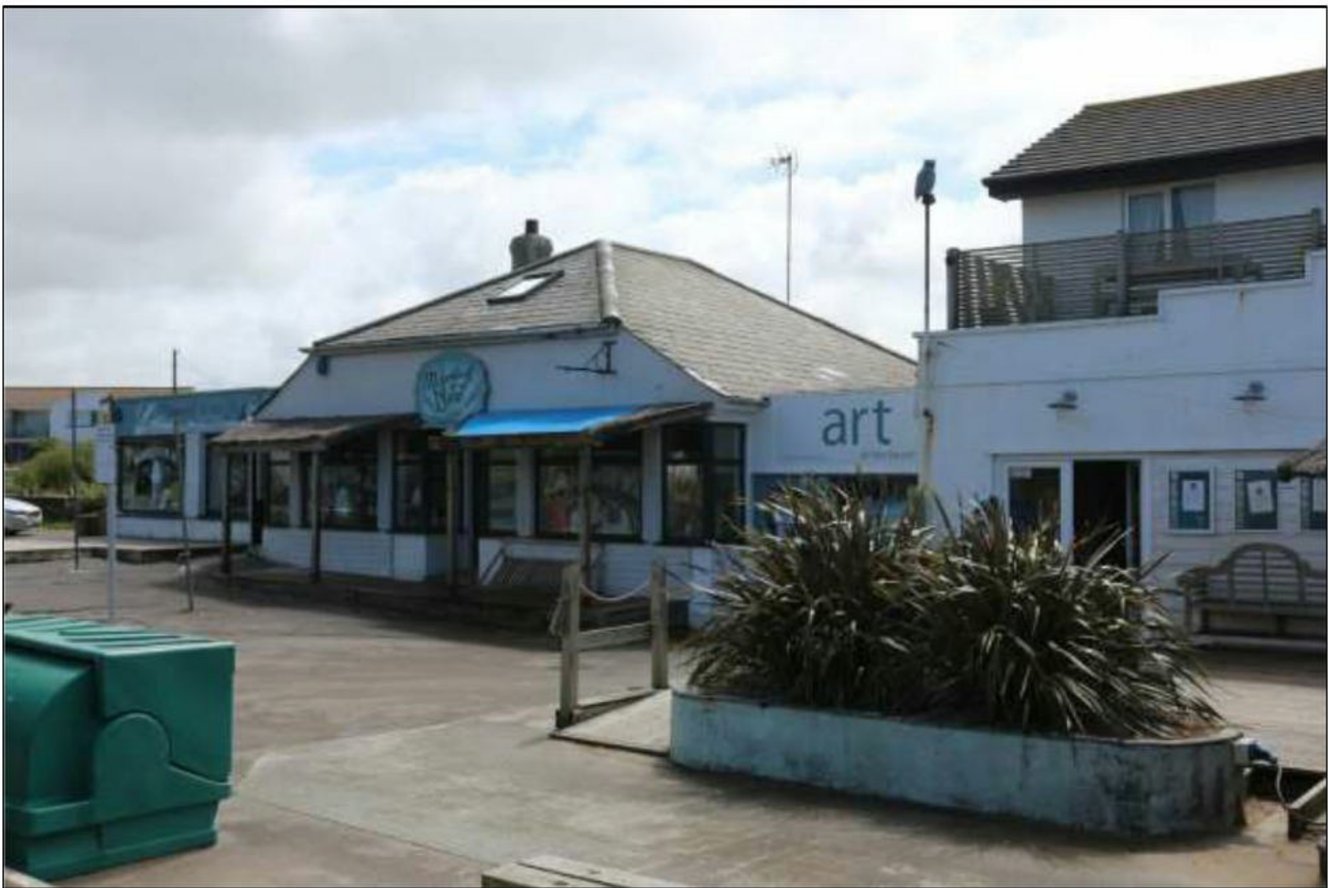
12. BUILDING 2, VIEWED FROM THE WEST.
