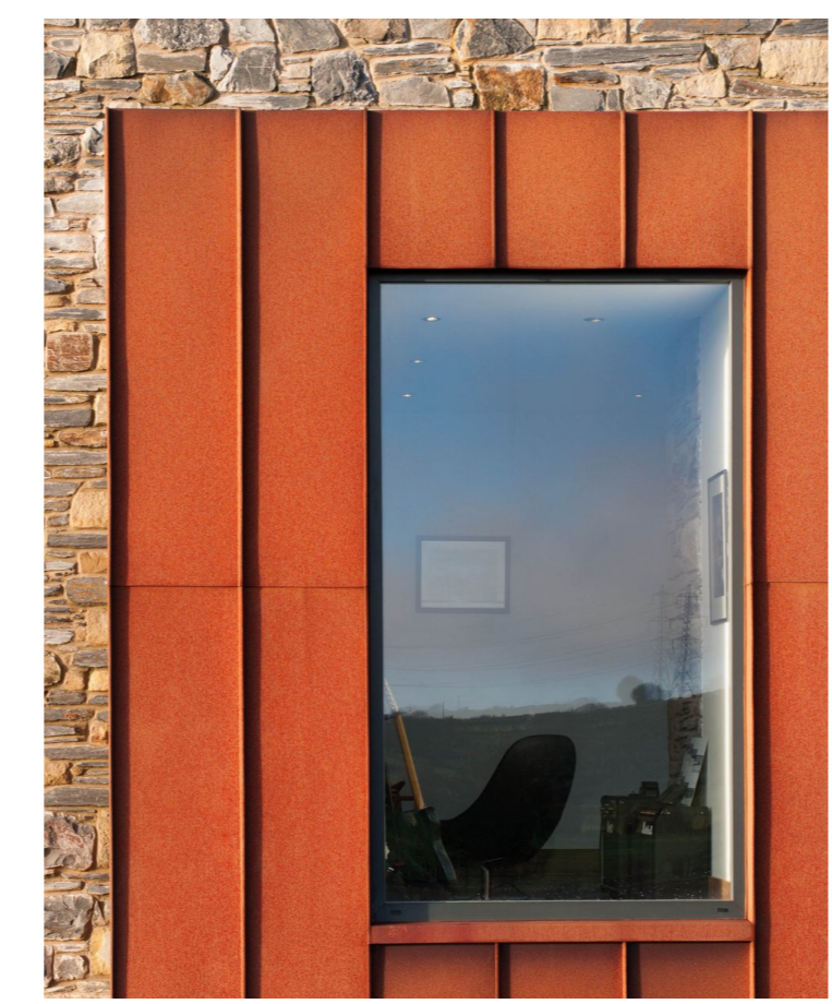
Precedent: Corten steel cladding
