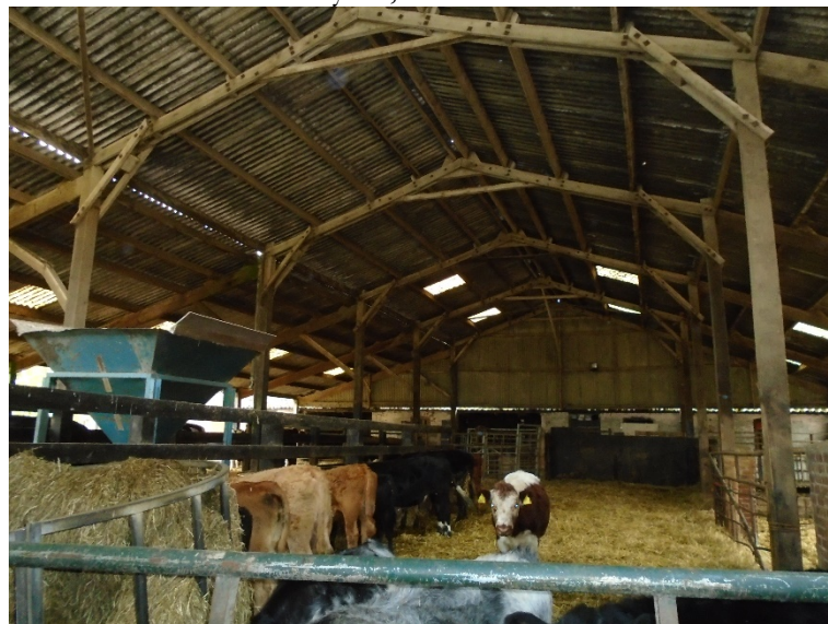
Plate 8 – fold yard, internal roof structure
