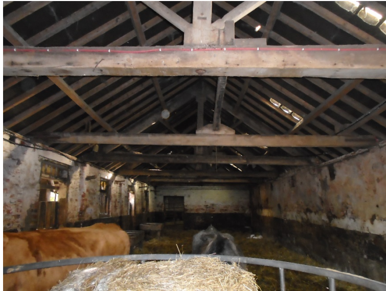
Plate 4 – barn 1, internal roof void
