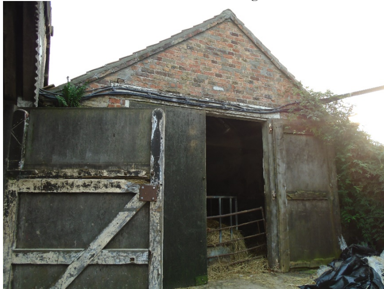
Plate 2 – barn 1, south gable
