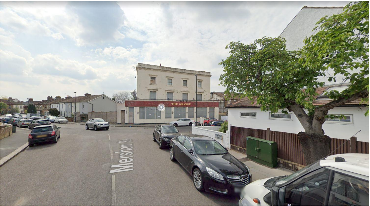
Fig 2. Front elevation viewed from Mersham Road.
