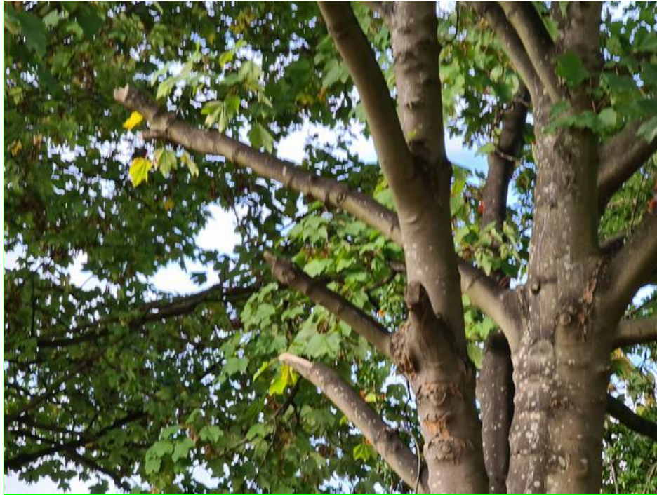
Image 7 Branche son the owner's side of T1 have been previously hacked back, see stubs
