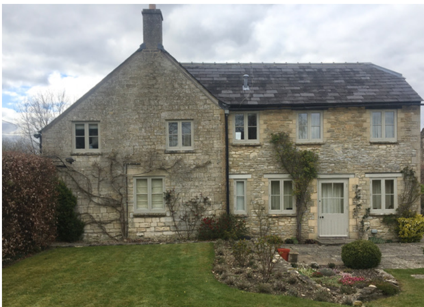
Photograph 1 - East elevation showing location of new door
