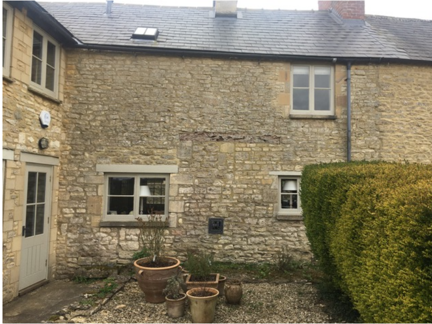
Photograph 2 - North elevation showing site of proposed extension
