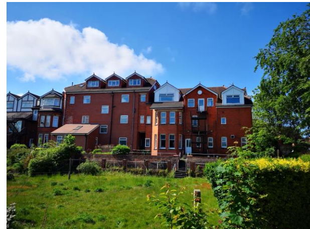
Rear view of existing nursing home
