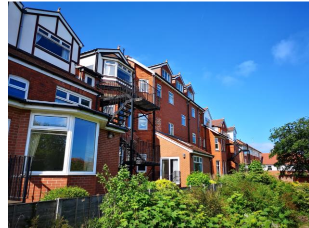
Rear view of existing nursing home
