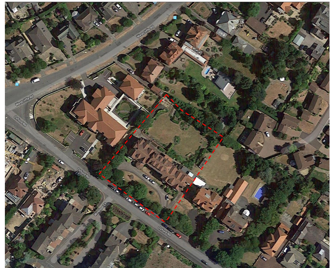
Ariel View of site as existing
