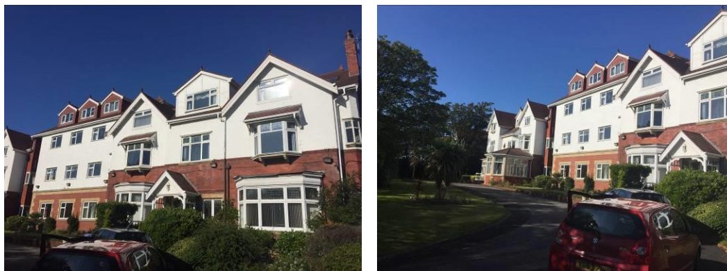
Plate 1: Front elevation of the property at 15-17 Oxford Road
