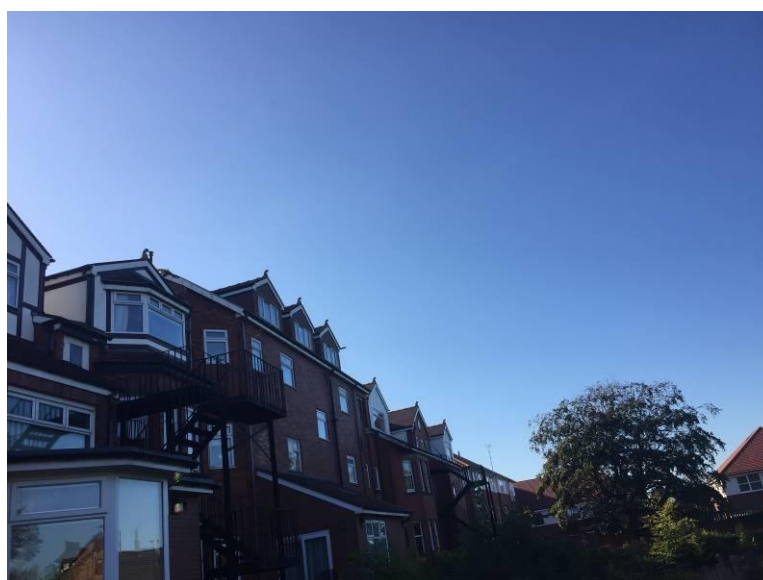
Plate 2: Rear elevation of the surveyed property
