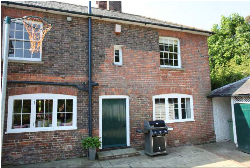
Plate 11: 19th century repair works to the rear cottage, facing southwest
