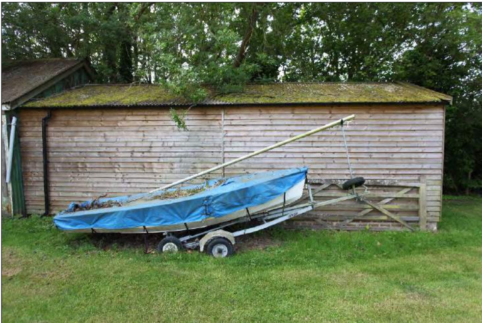
Plate 2: West range of timber outbuilding, facing south
