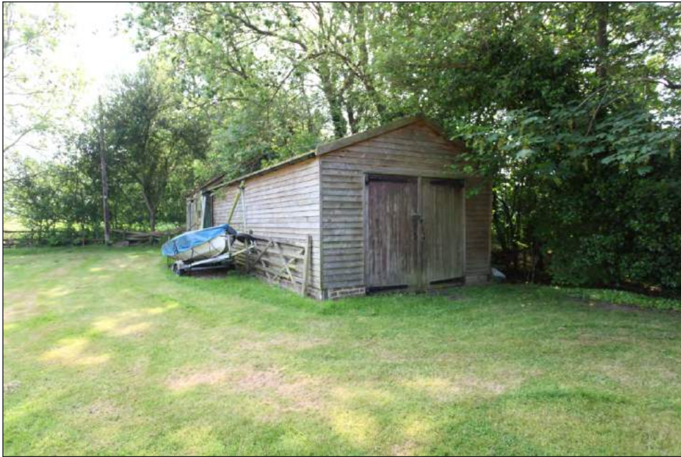
Plate 3: View of timber outbuilding, facing southeast
