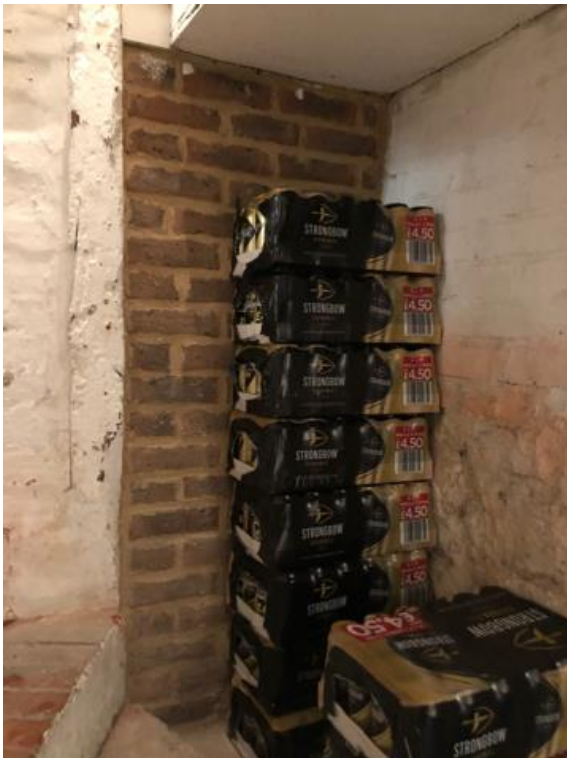
Bricked up door on shop side (35)
