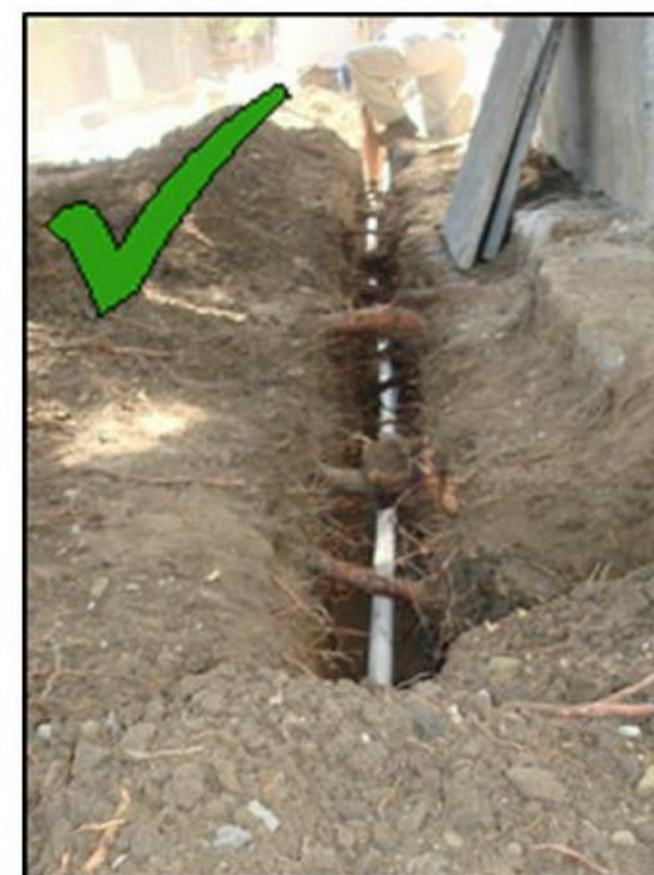
Significant roots retained
