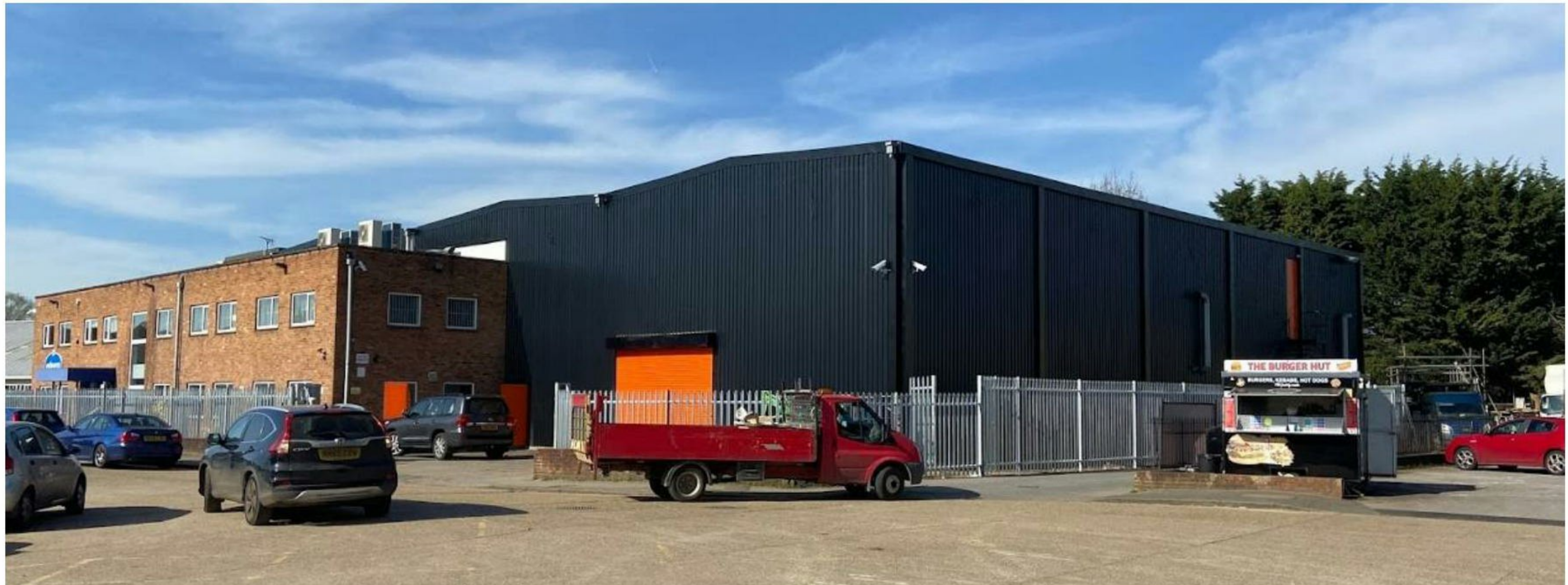
Photo 2 – Unit after recladding
