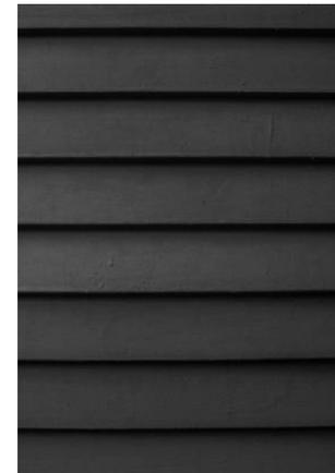
Above the brick, the remainder of the walls will be clad in timber weatherboard painted black; typical of Kentish agricultural buildings.
