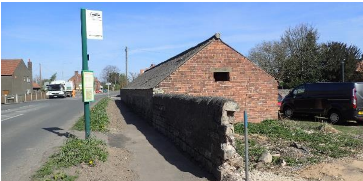
Photograph 3: South gable and west aspect of Barn 4
