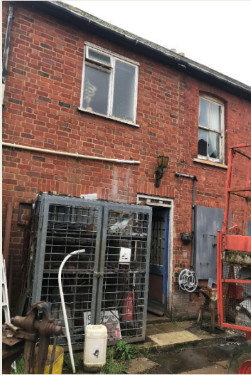
The house in the north west.
