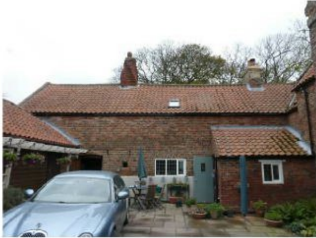
Courtyard Elevation Blacksmiths Forge to left
