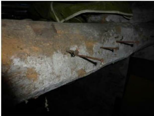
Blacksmiths Forge existing first floor beam to be retained
