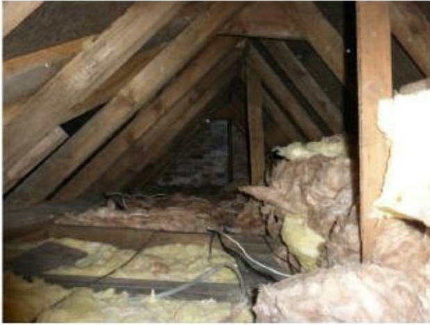
Roof void above new bedroom
