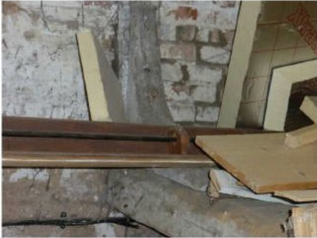
Blacksmiths Forge interior. Mezzanine position Unusual, inverted knee brace to beam ends
