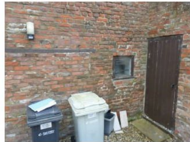
Blacksmiths Forge. Main entrance area.
