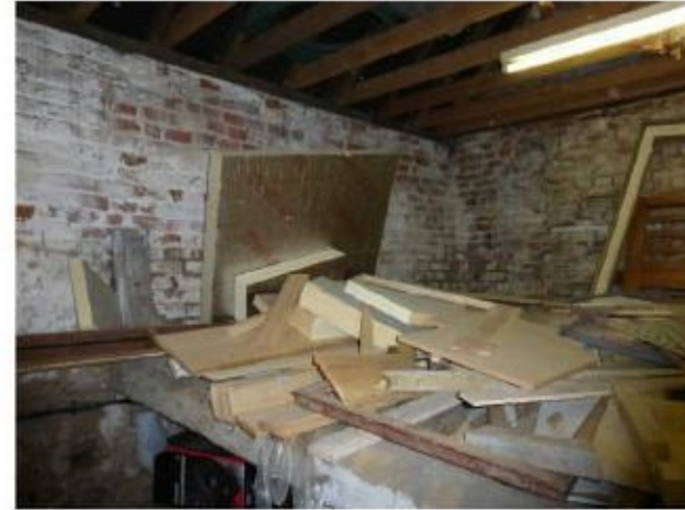
Blacksmiths Forge existing first floor.
