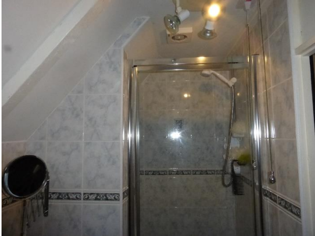
First Floor Area existing shower room
