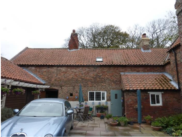
Courtyard Elevation Blacksmiths Forge to left
