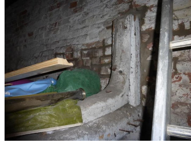
Blacksmiths Forge existing first floor beam to be retained Unusual, inverted knee brace to beam ends
