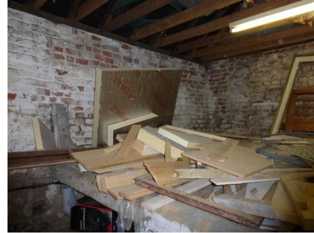
Blacksmiths Forge existing first floor.
