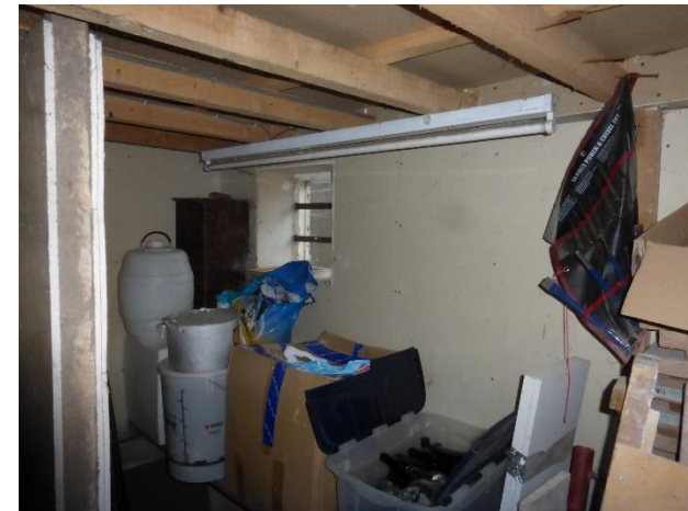
Blacksmiths Forge interior
