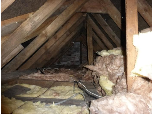
Roof void above new bedroom
