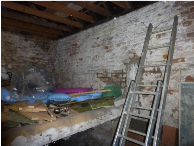
Blacksmiths Forge existing first floor.
