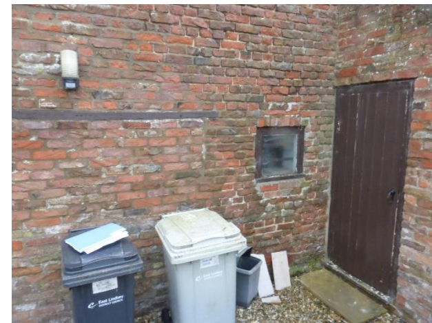
Blacksmiths Forge. Main entrance area.
