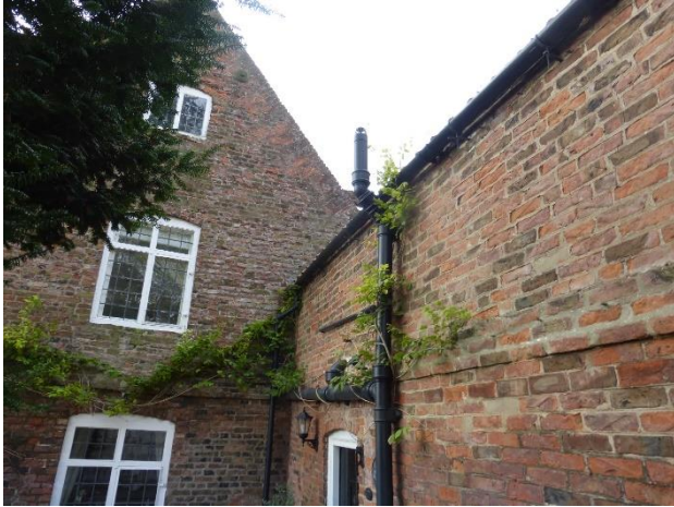
Main Entrance to Guest House
