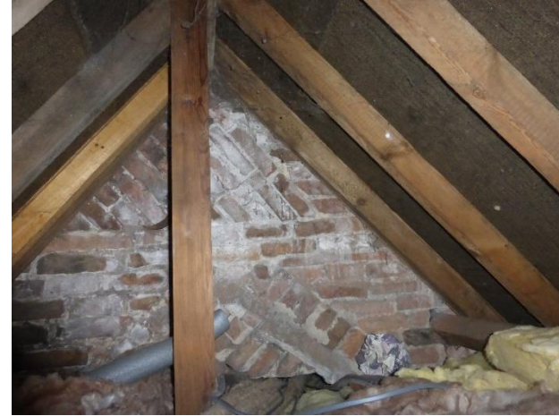
Roof void above new bedroom. Brick chimney stack with arch gathering
