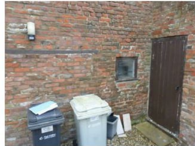
Blacksmiths Forge. Main entrance area.
