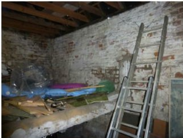
Blacksmiths Forge existing first floor.
