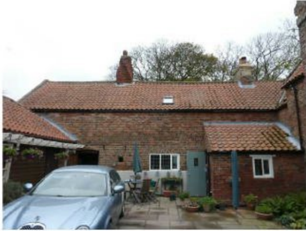
Courtyard Elevation Blacksmiths Forge to left
