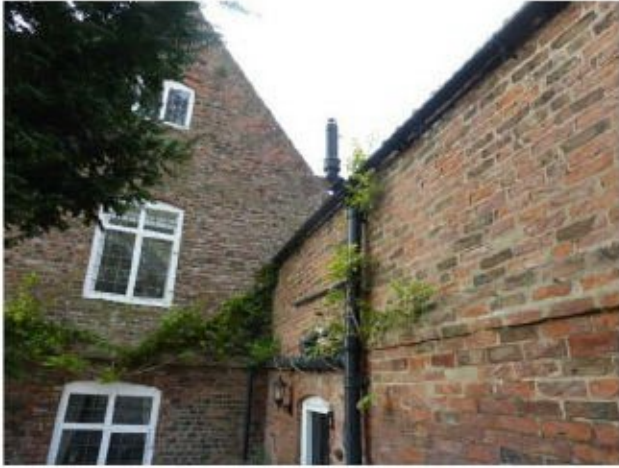
Main Entrance to Guest House
