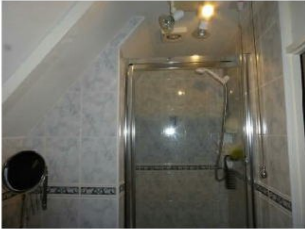
First Floor Area existing shower room
