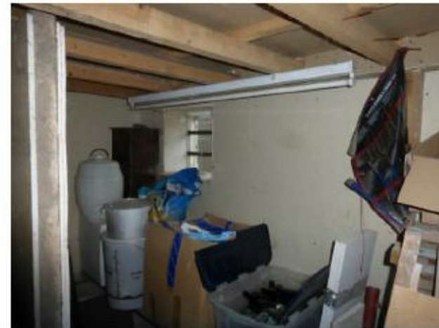
Blacksmiths Forge interior
