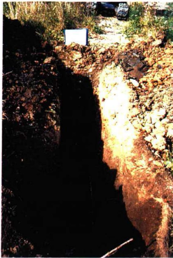
Plate 1 – Excavation of TP19
