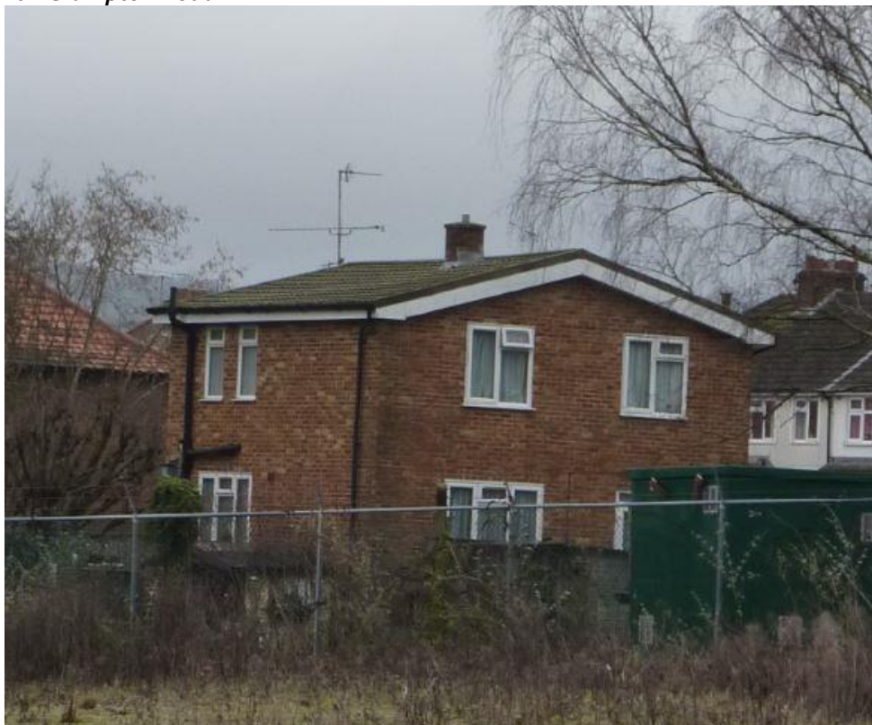
Image 7 - Rear and flank façade of 107 Crampton Road
