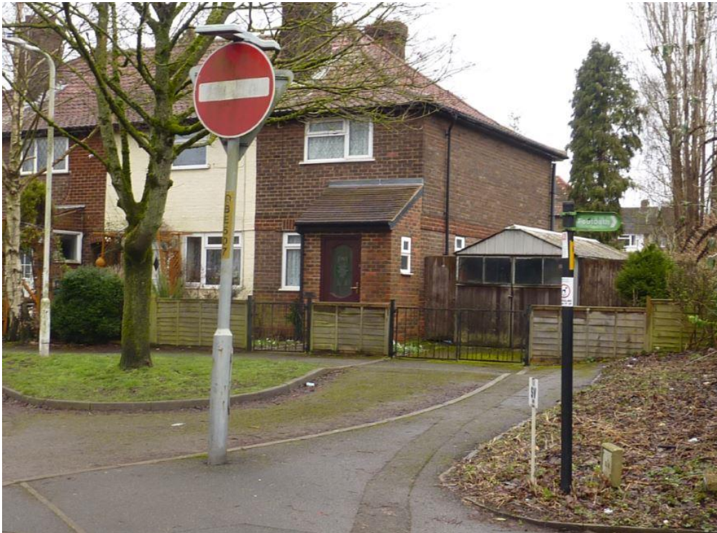
Image 3 - Front and flank facades of 114 Otford Road
