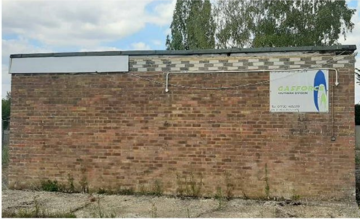
Plate 9.1: Building with Bat Potential
