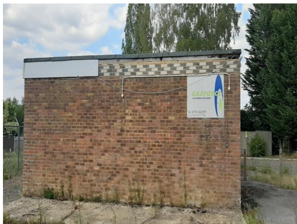
Plate 4.1: Building B1 (Southern Elevation)
