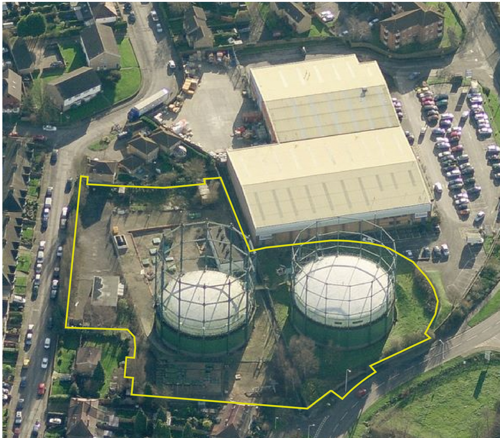
Birds eye view pre-demolition with application boundary line
