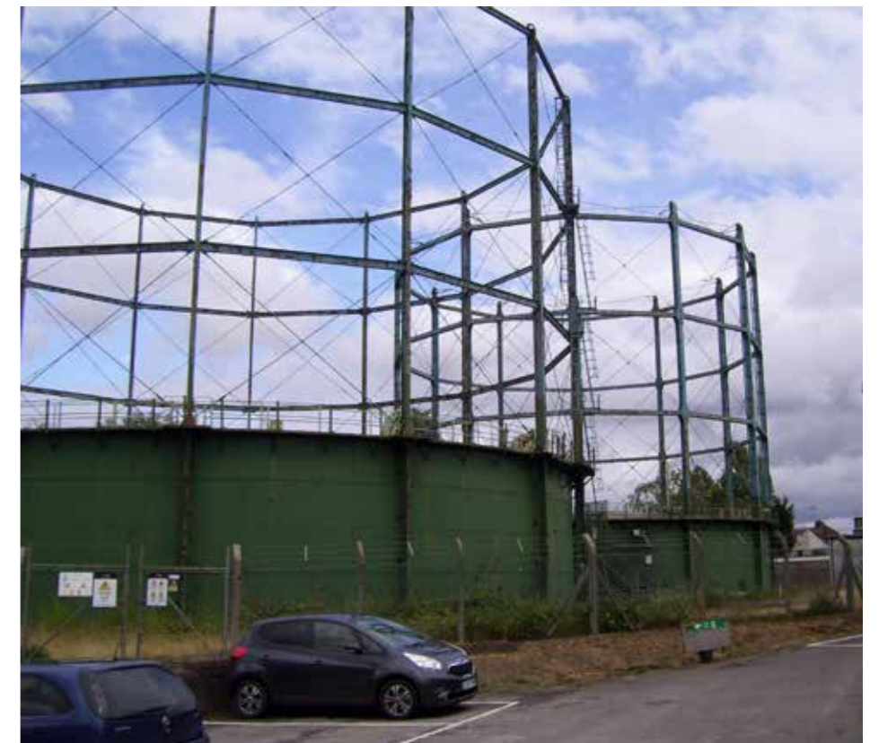
Historic photograph of gasholders before demolition
