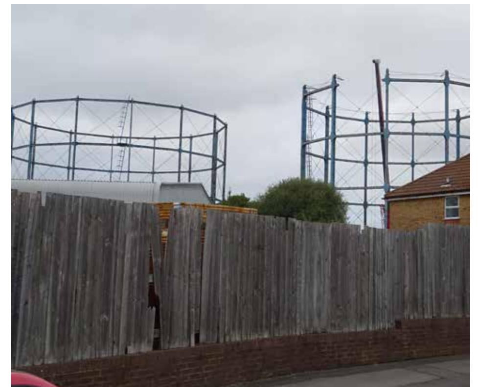
Historic photograph of gasholders being demolished
