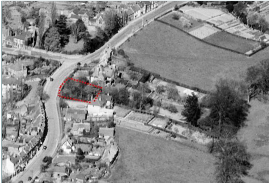
Plate 5. Aerial view of the Wantage. Taken in 1953. The site is densely planted
