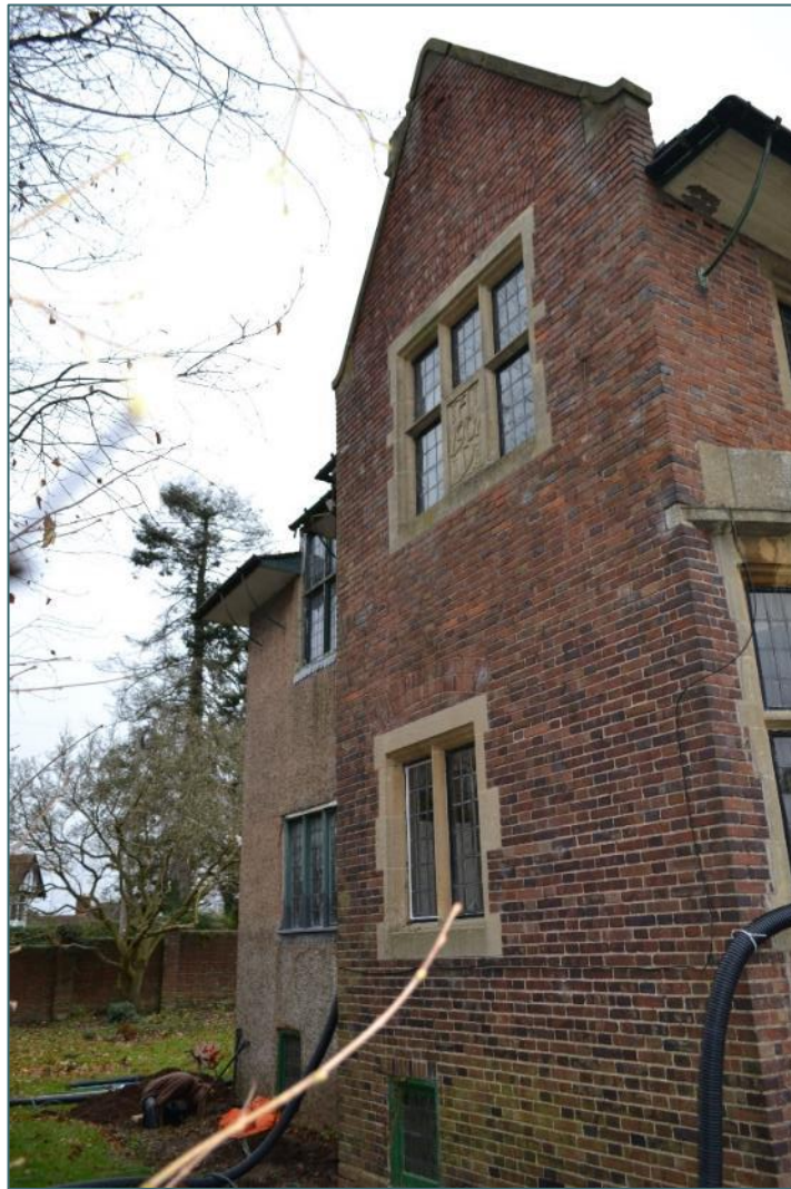
Photo 11. West elevation of 1 Castle Hill
