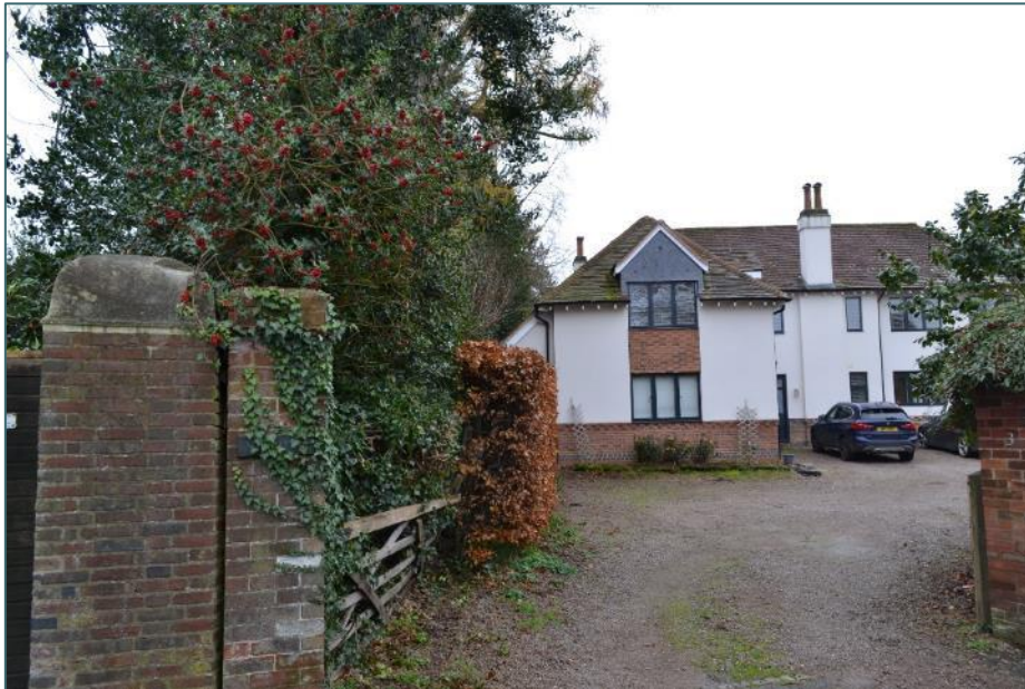
Photo 16. 3 Castle Hill. The brick pier on the left belongs to 1 Castle Hill
