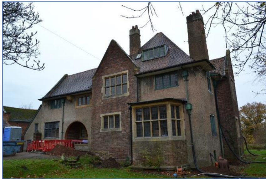
Photo 9. North elevation of 1 Castle Hill
