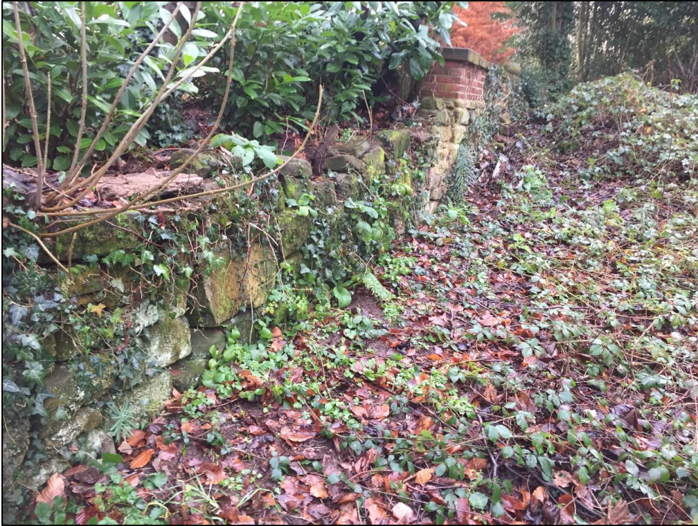
Photograph 2 east boundary wall
