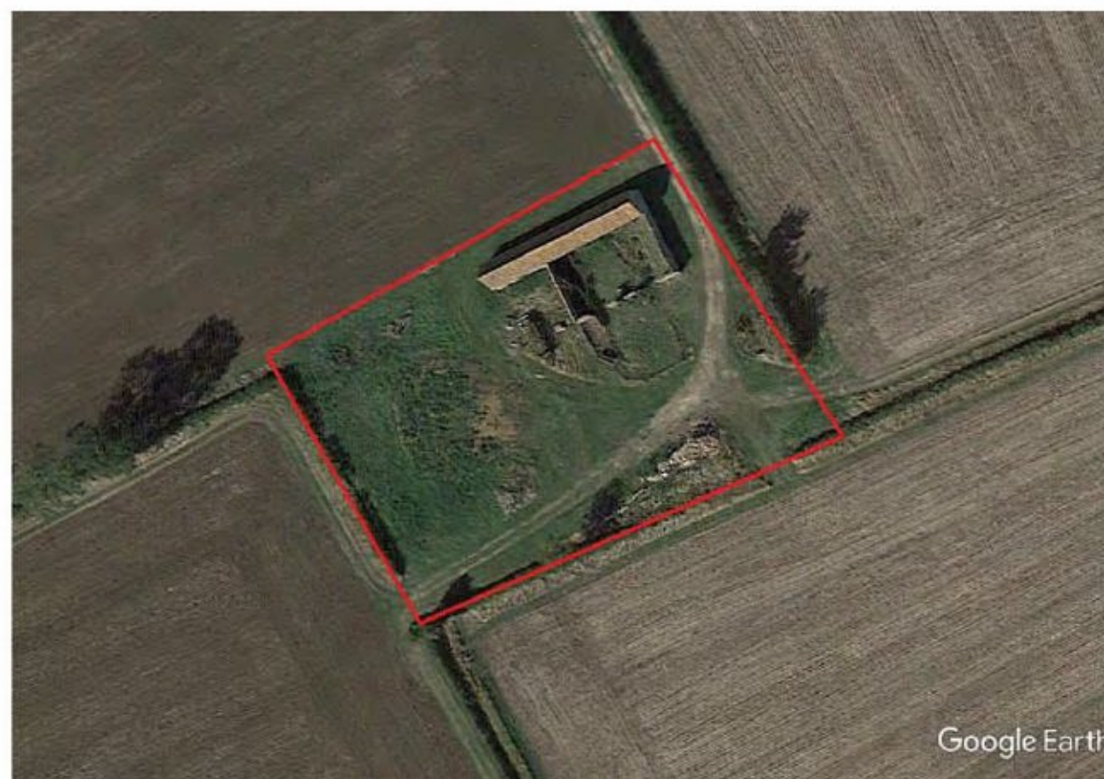
Figure 1: Aerial view of the survey site, outlined in red
