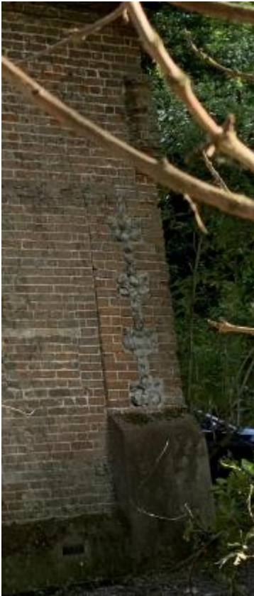
North west corner showing a vertical break in the coursing where later brickwork abuts the West gable
