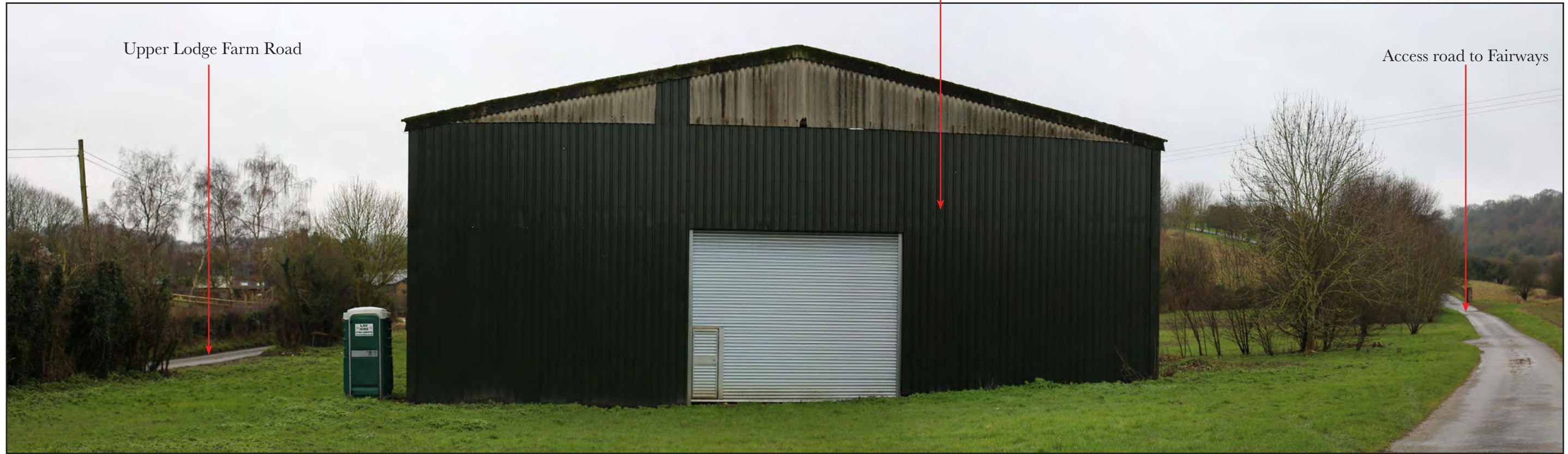
Photoview 1 - View looking south
