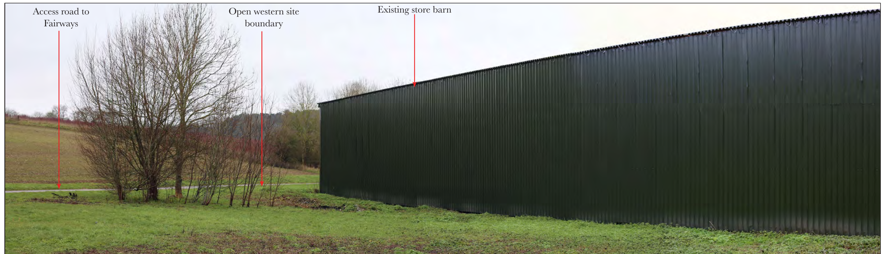
Photoview 6 - View from the site entrance looking north-east
