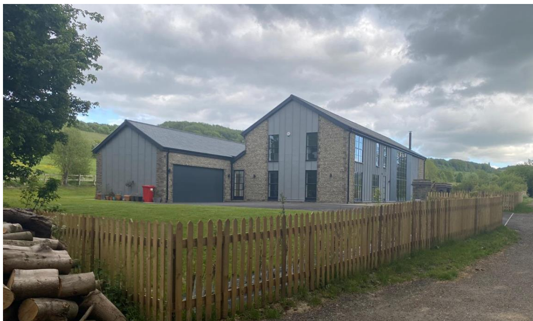
Recently completed development at Austin Lodge
