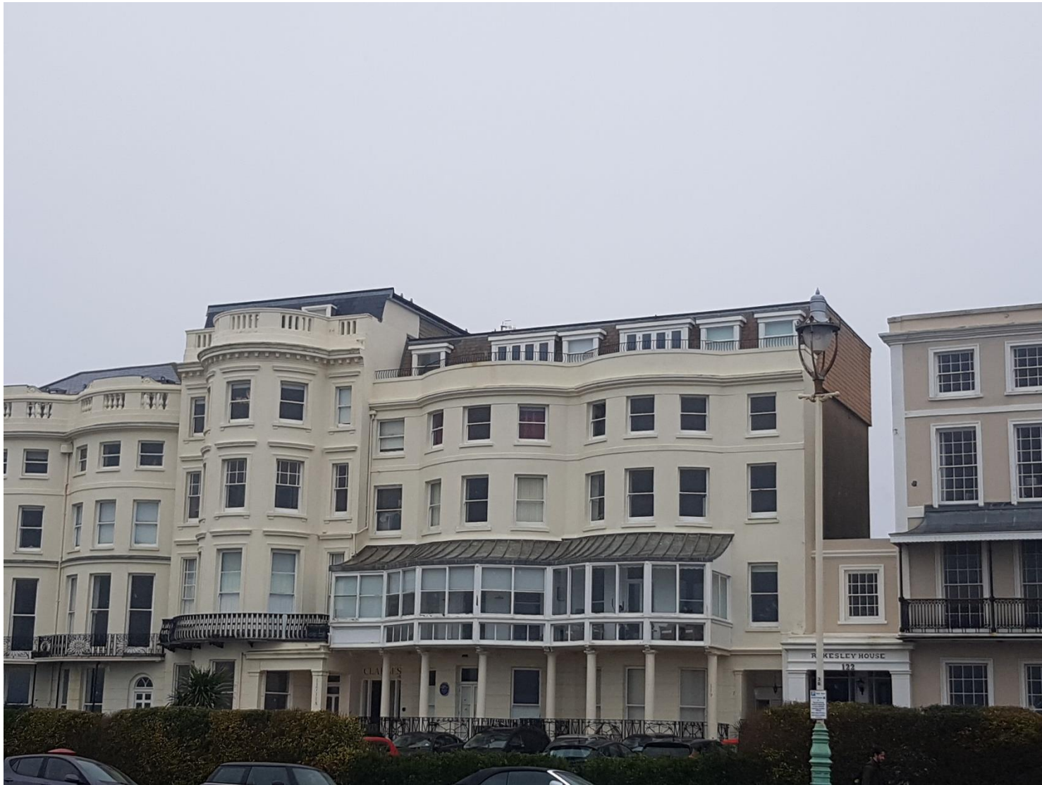
4 Angled view of Flat 16 (Penthouse)
