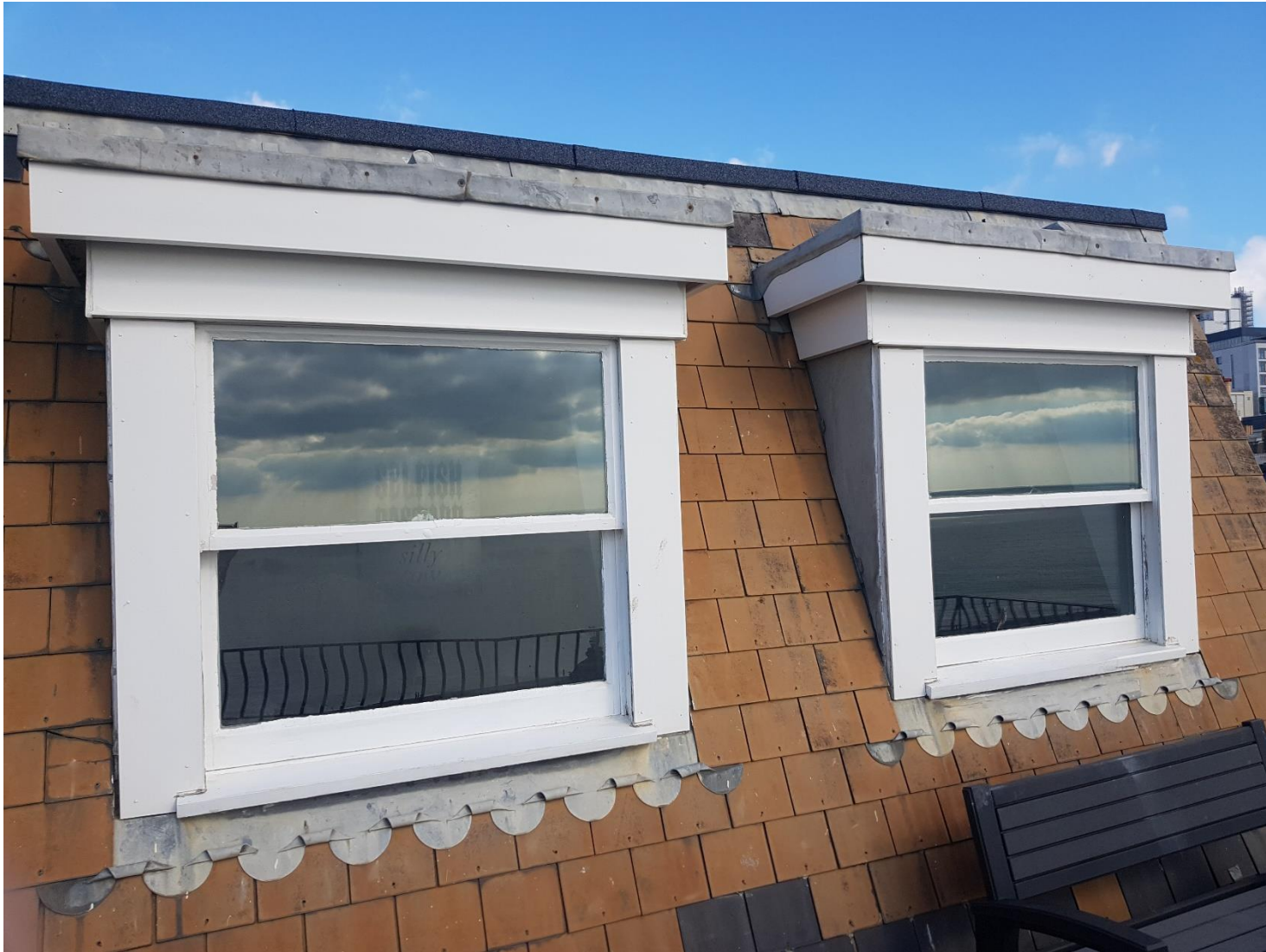
7 Closer view of typical South elevation windows
