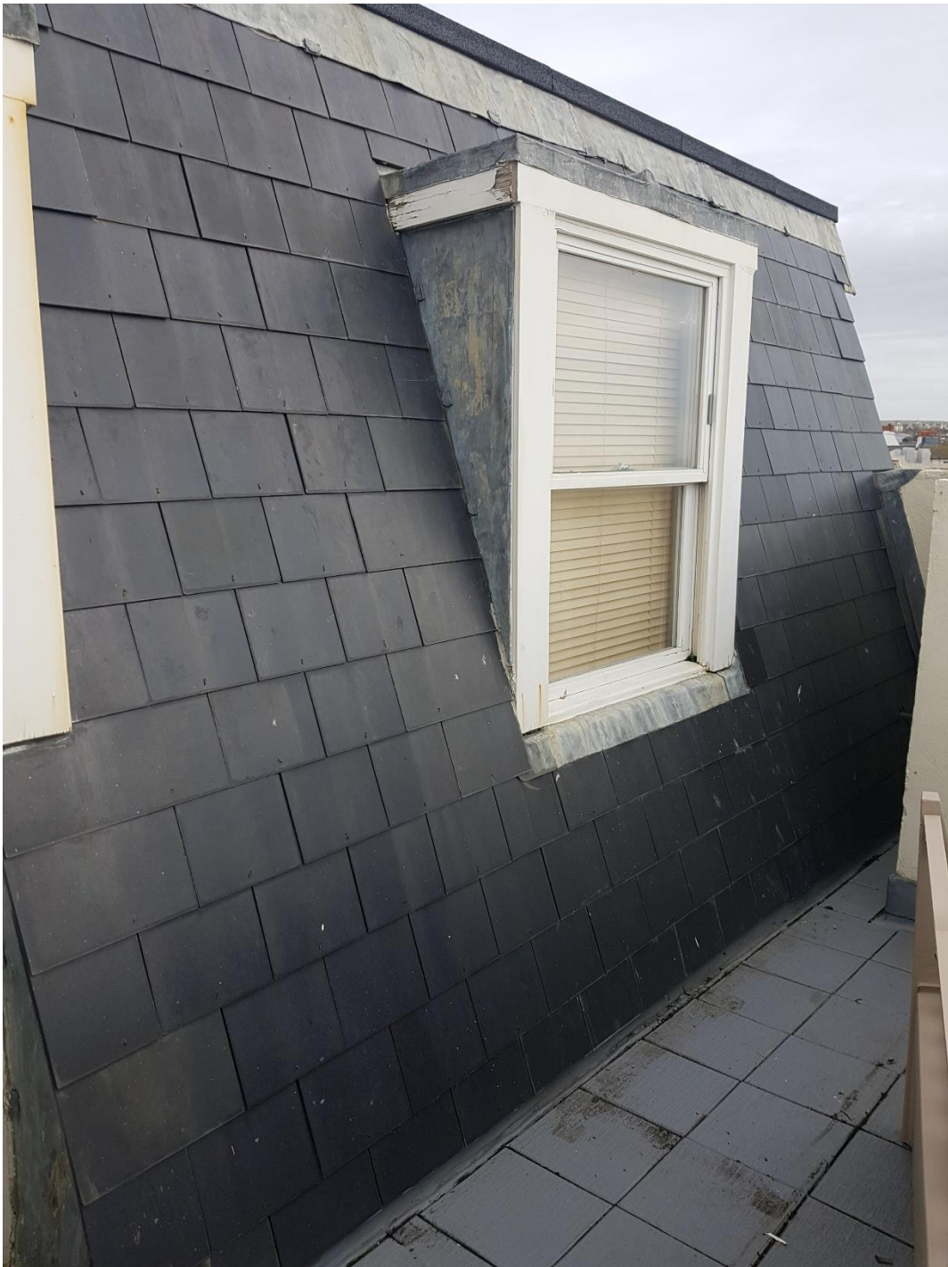
6 View of Tiles and Window - upper section (West side)
