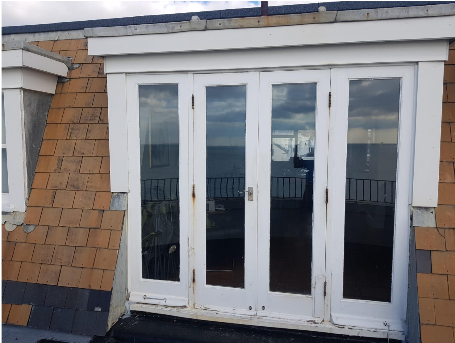
8 Close view of a typical door on south elevation
