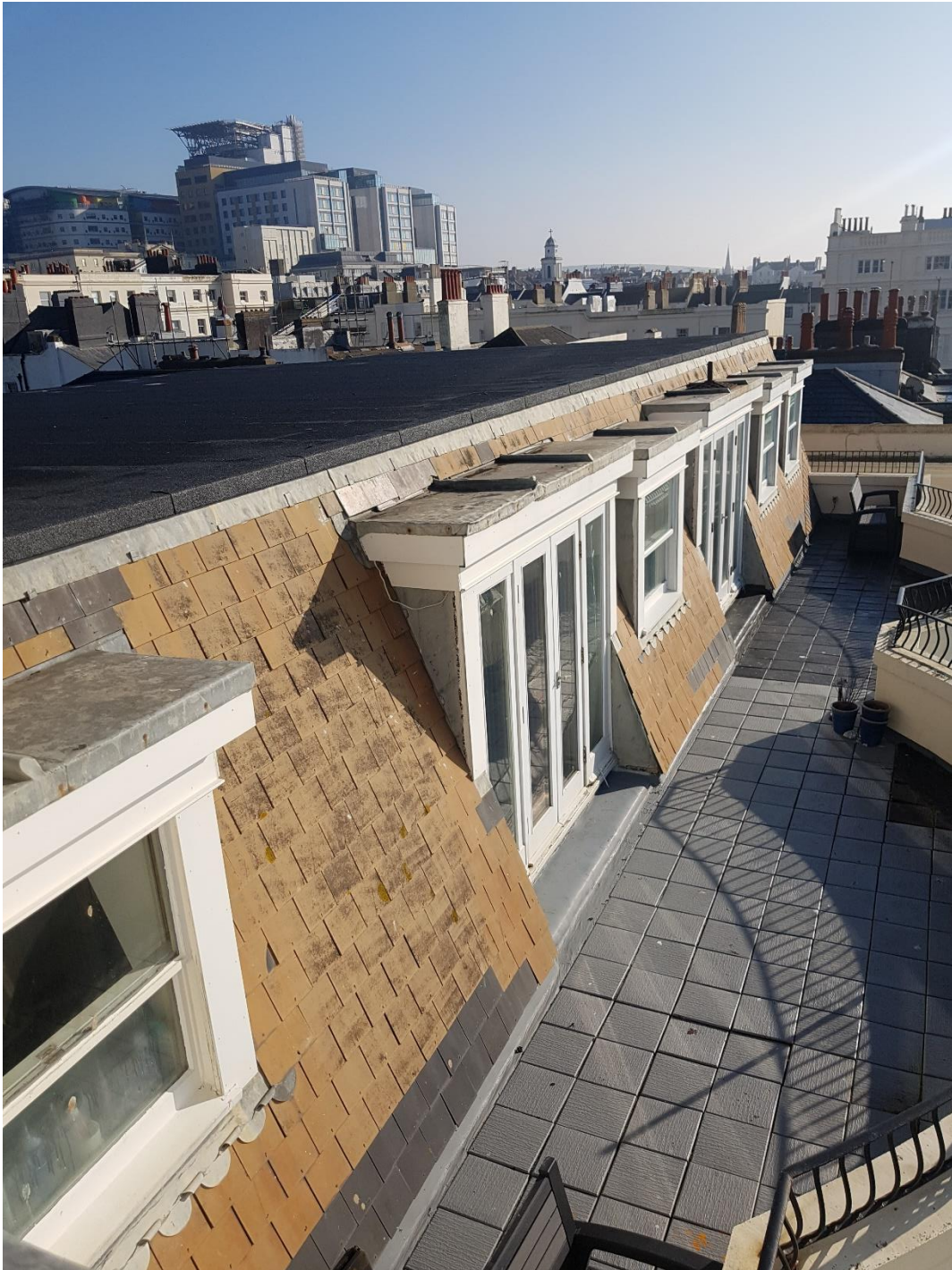
5 View of; Tiles, Windows and doors - lower section (East side)
