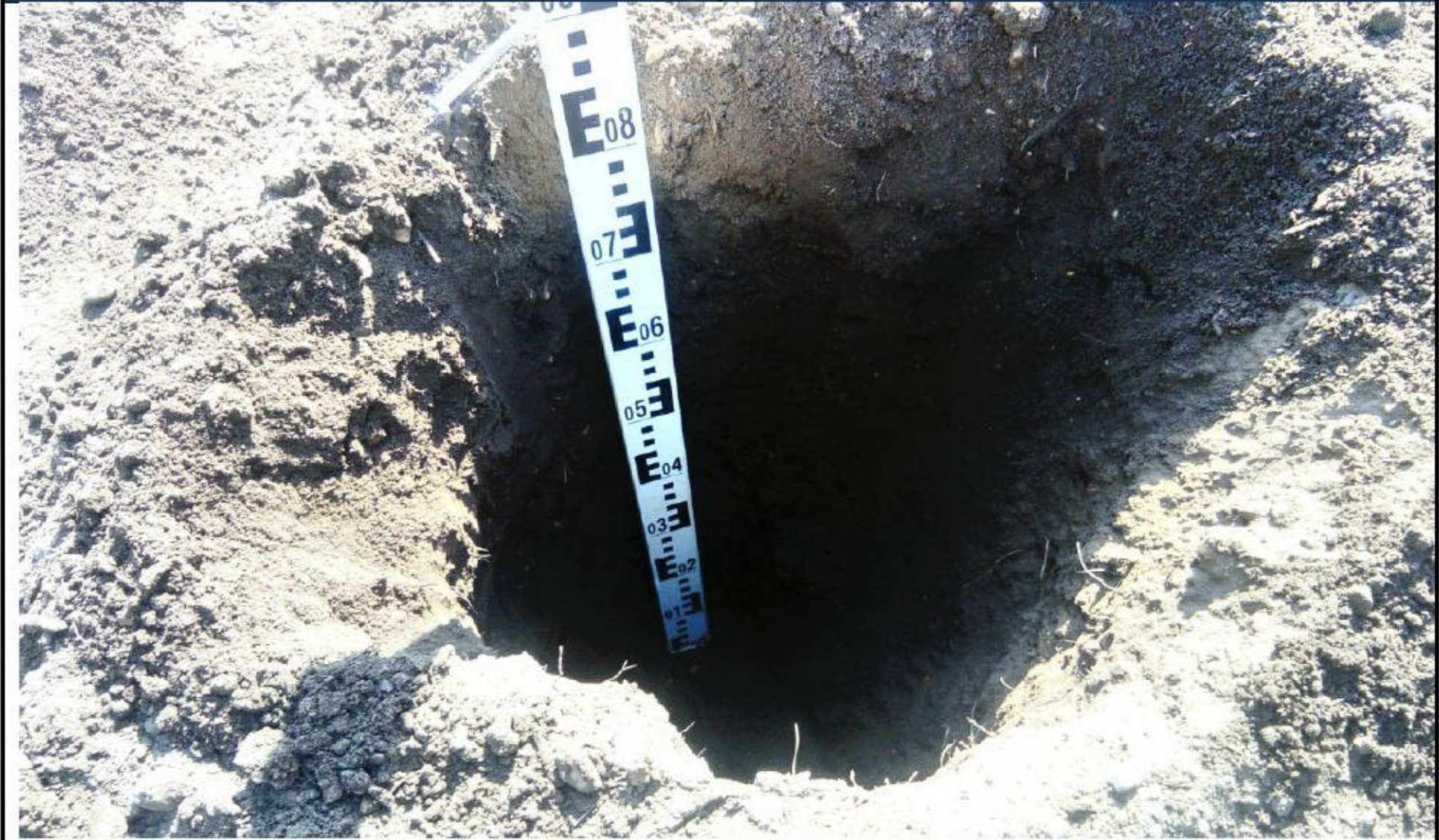
Plot 25 hand excavated pit
