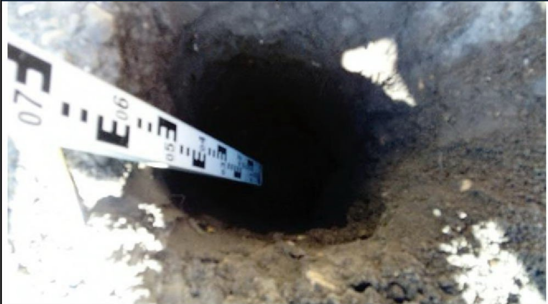
Plot 26 hand excavated pit
