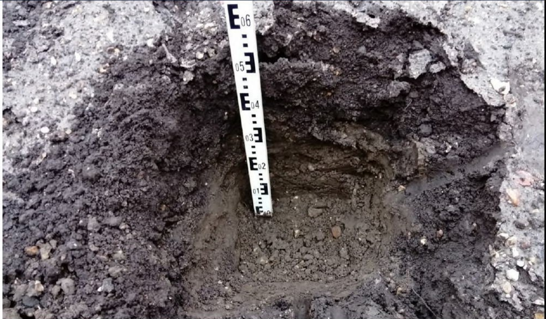
Plot 29 hand excavated pit
