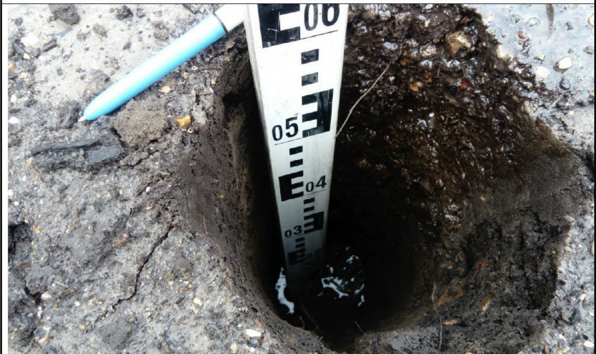
Plot 29B hand excavated pit
