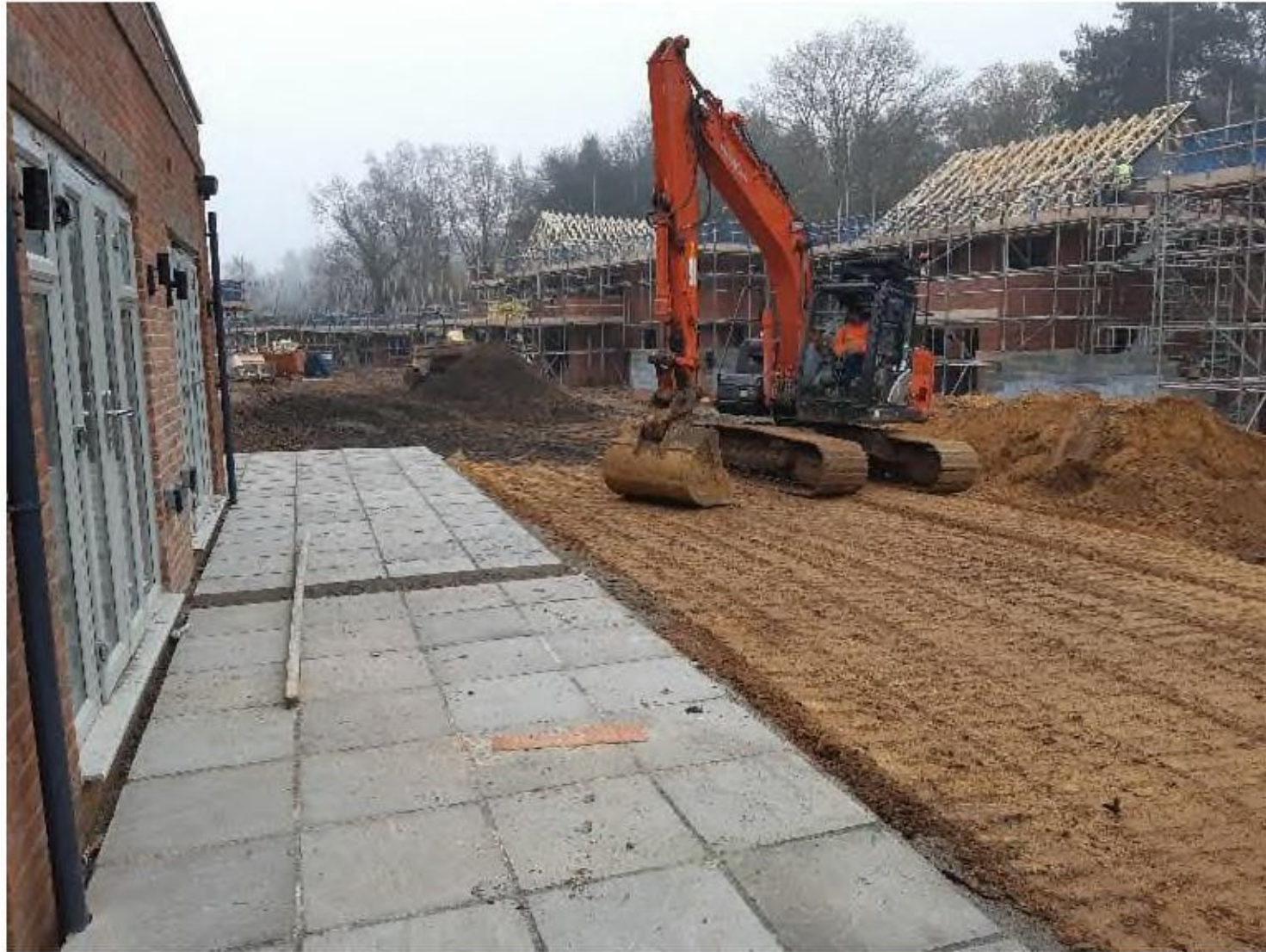
Tracking placed topsoil in Plot 184 + 185.
