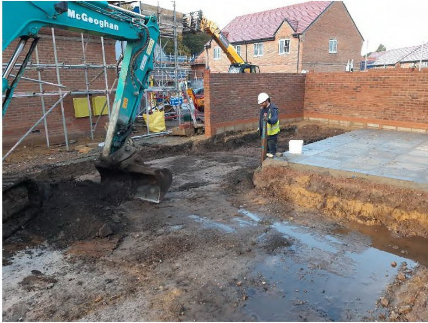
Excavating to formation level in Plot 178 and 179.
