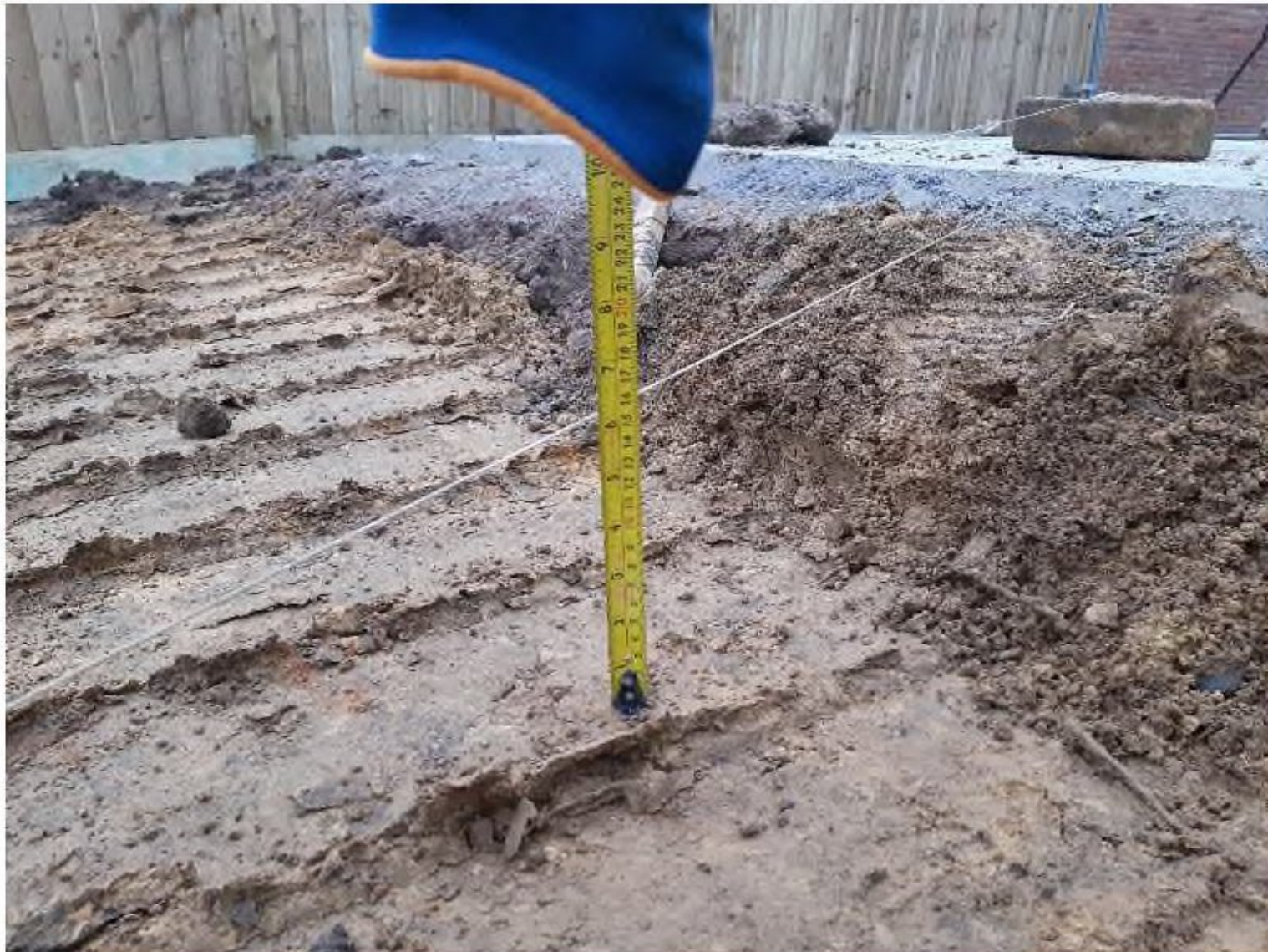
Space left for topsoil in Plots 184 + 185.
