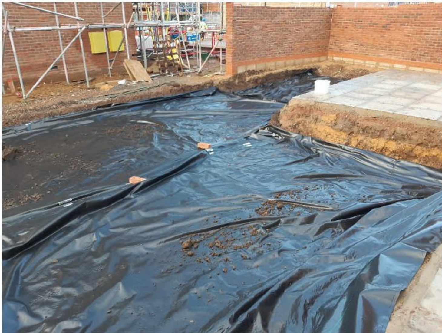
Membrane at formation level in Plots 178 and 179.
