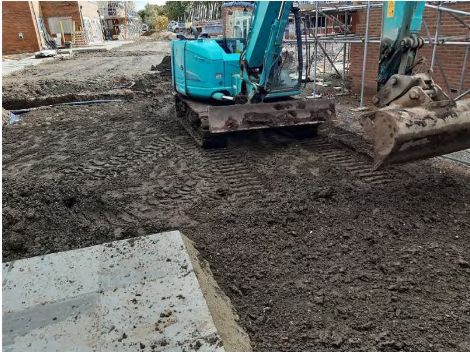
Placing of subsoil in layers in Plots 178 and 179.
