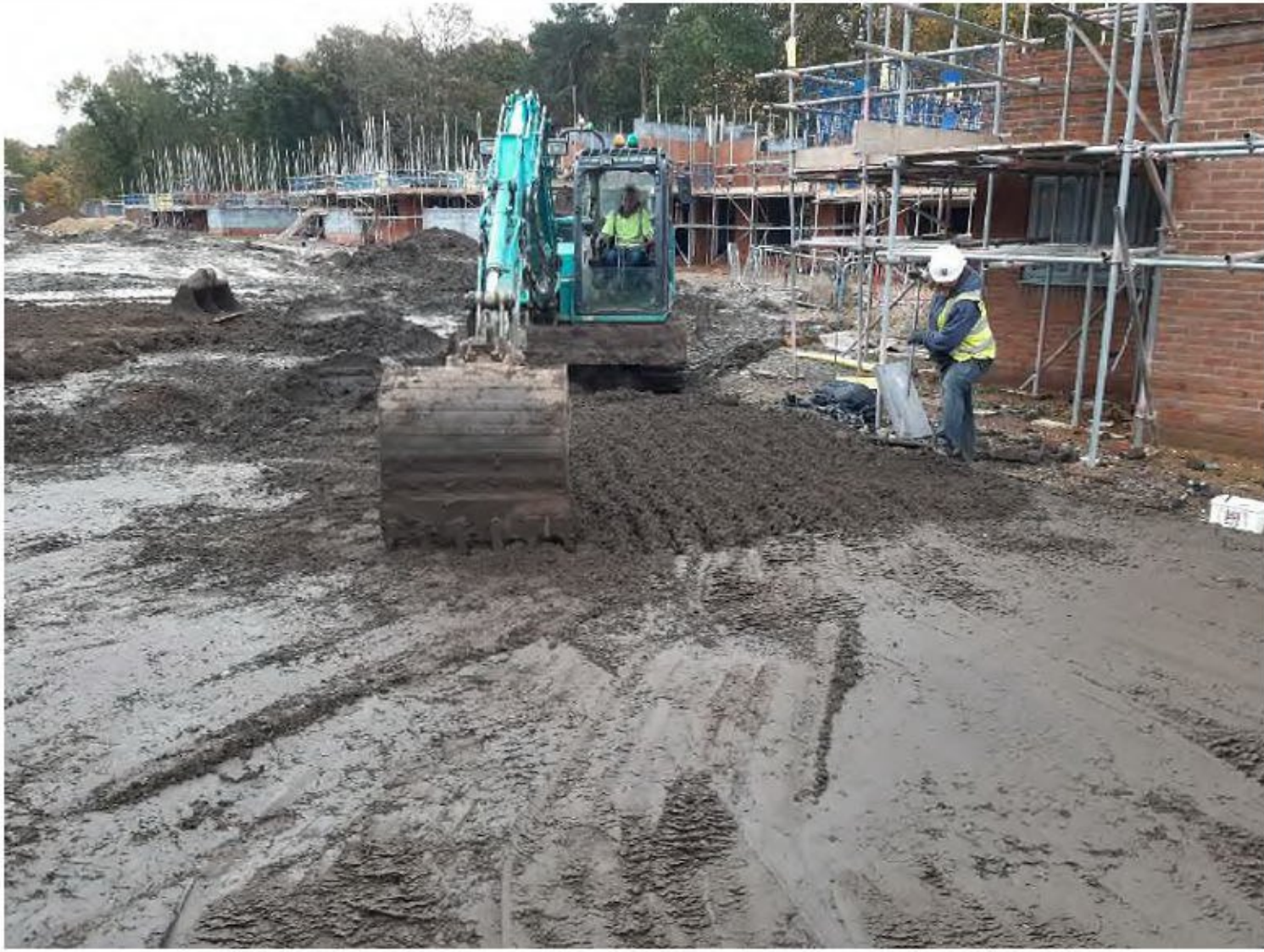
Raking placed topsoil with excavator bucket for picking in Plot 178.
