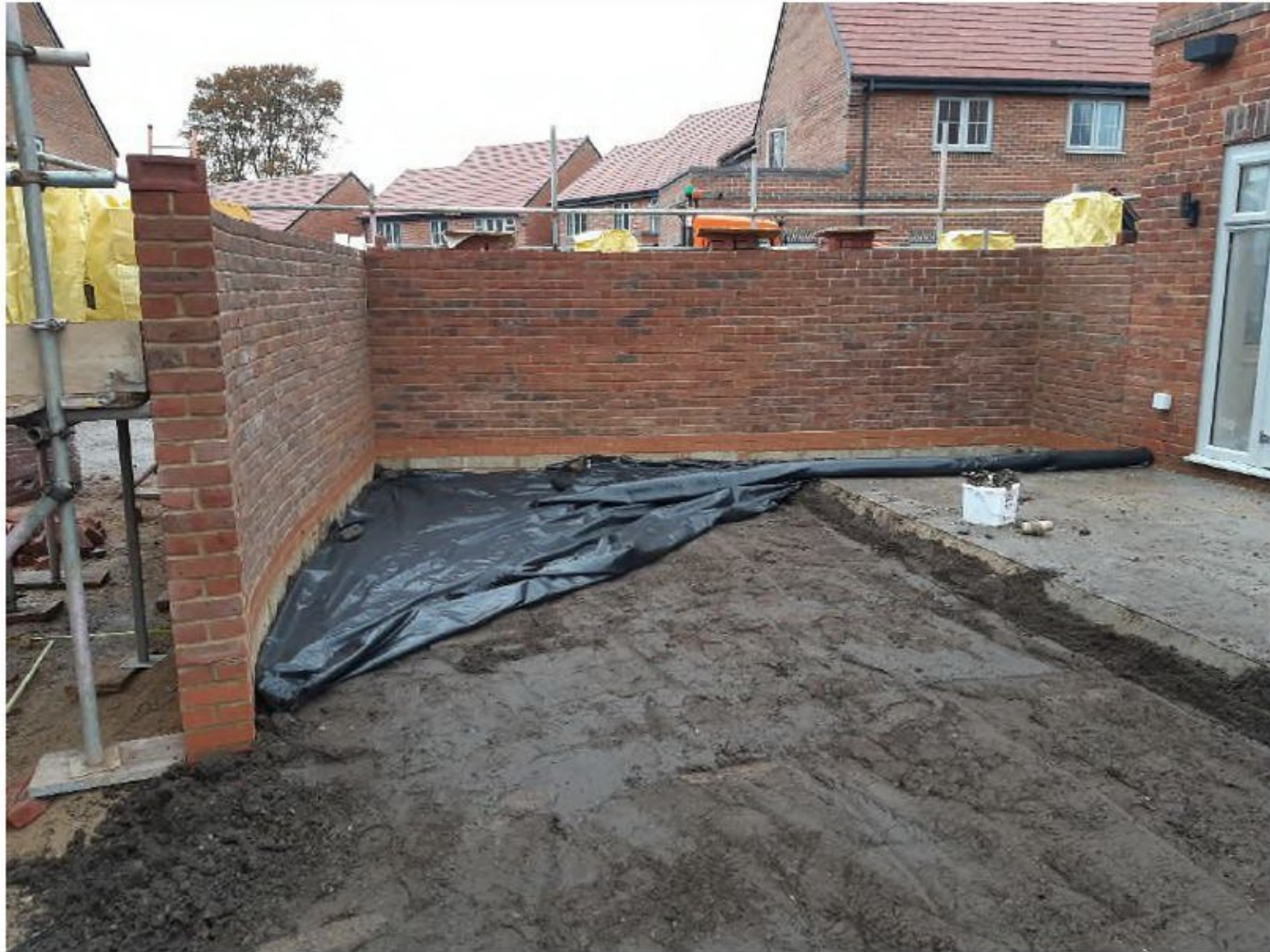
Protection measures from follow on trades in Plot 178.
