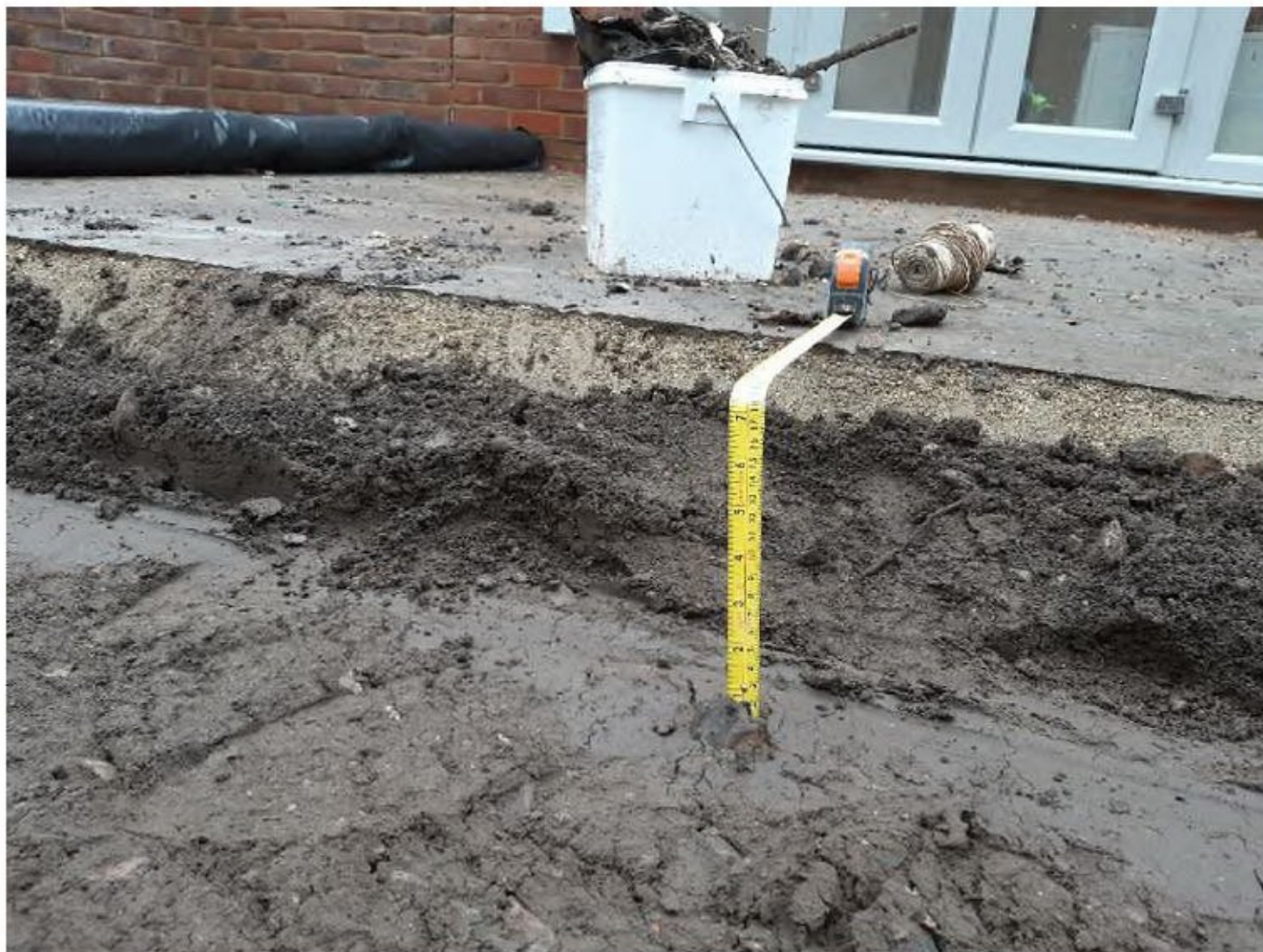
Space left for topsoil in Plots 178 and 179.
