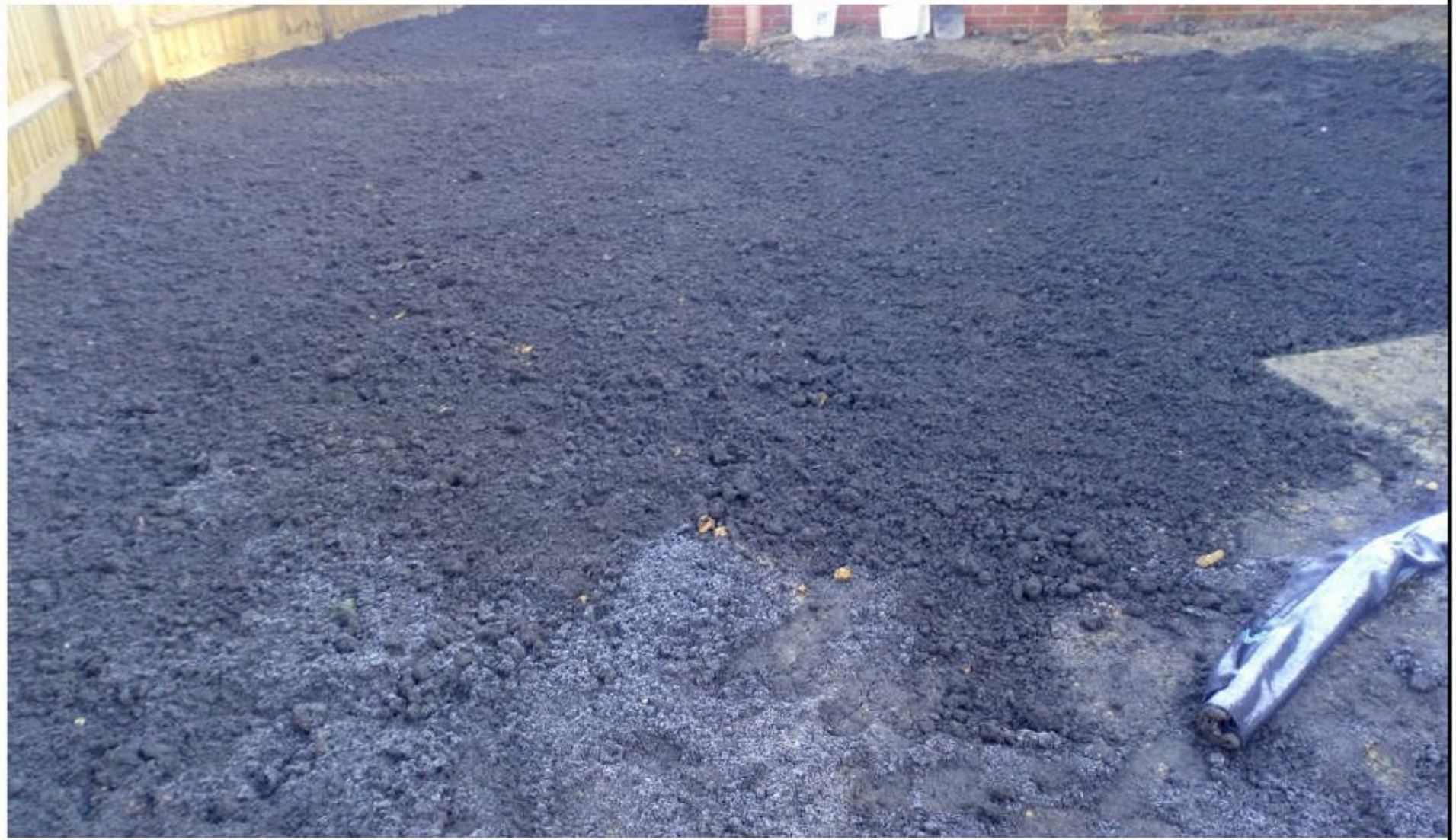
Topsoil completed in Plot 177
