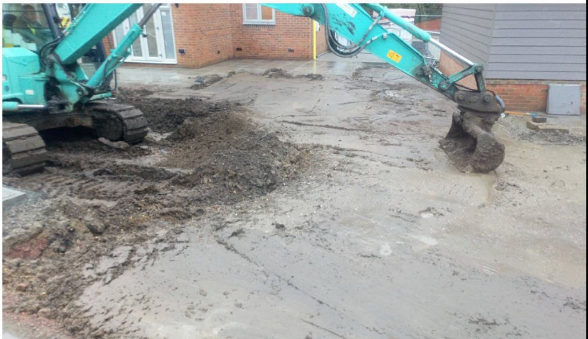
Placement of subsoil on membrane for Plot 174
