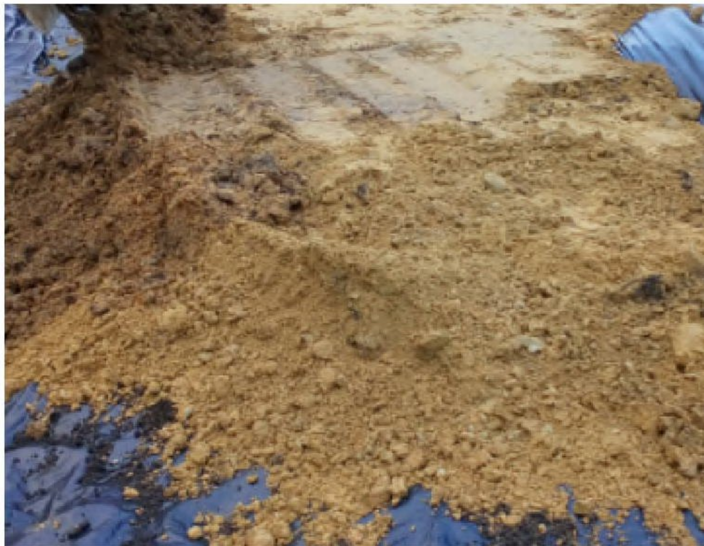
Placement of subsoil in Plot 177
