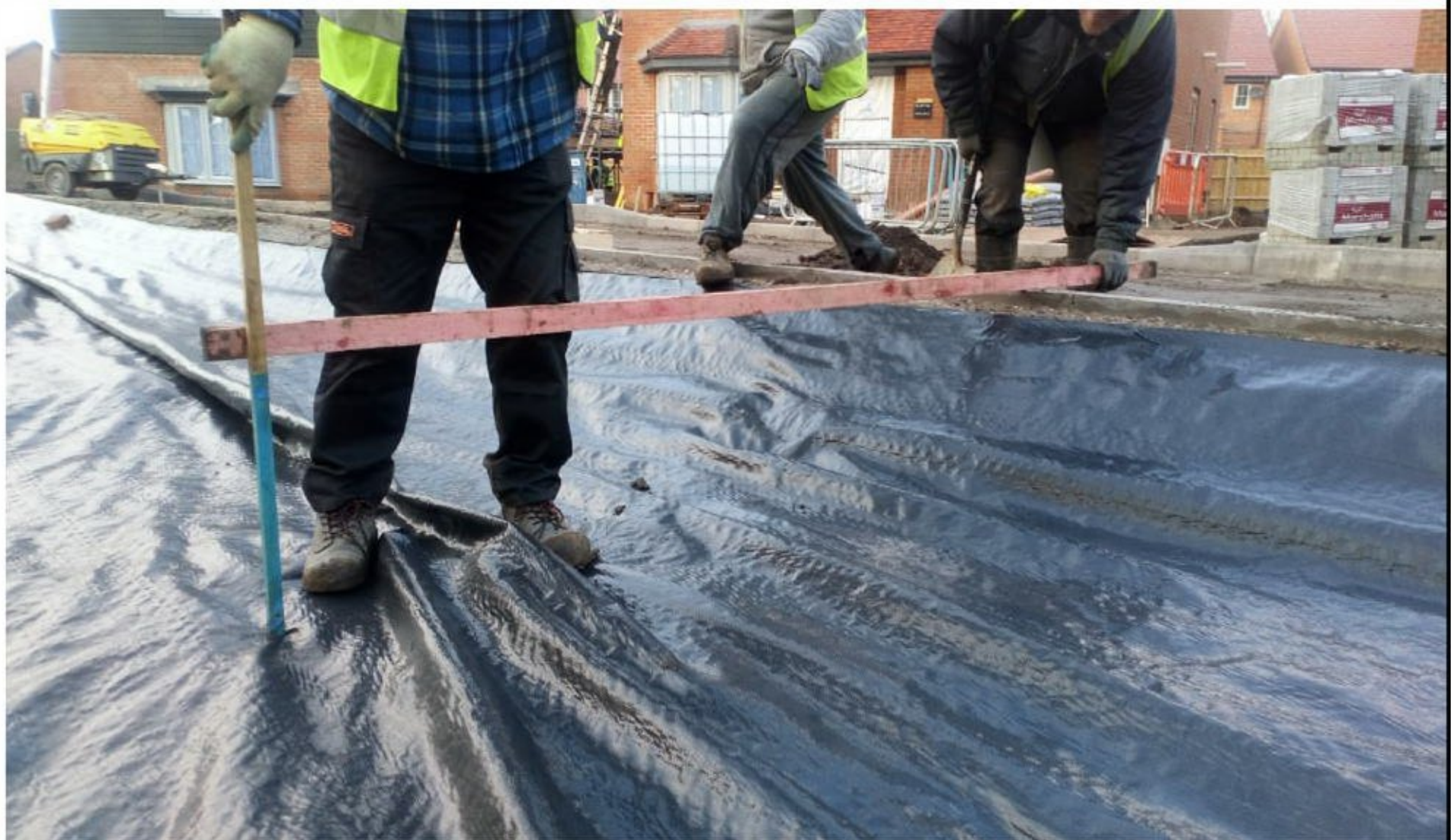
Placement of membrane and measuring depth to 600mm
