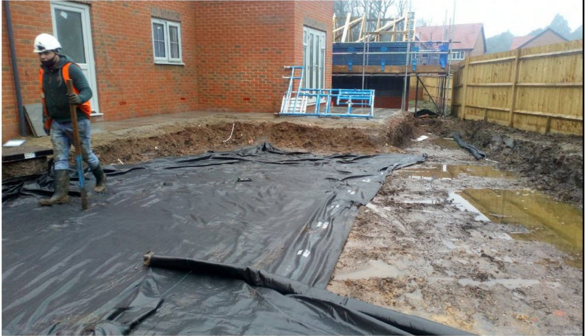
Placement of membrane in Plots 175 and 176
