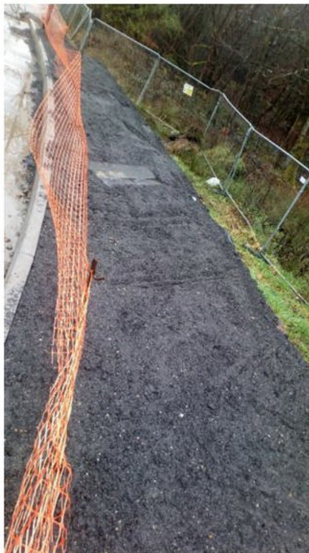
POS finished with Topsoil
