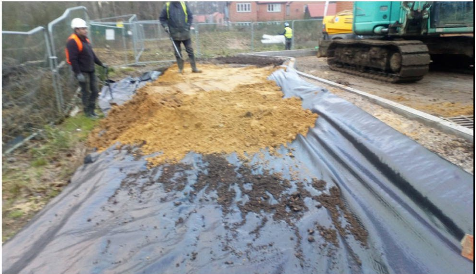
Membrane with layer of subsoil on
