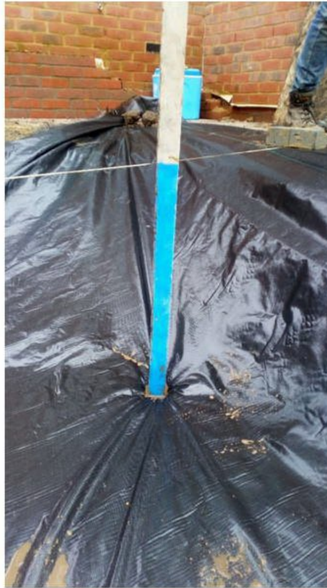
Laying and placement of membrane and formation measuring depth in Plot 177
