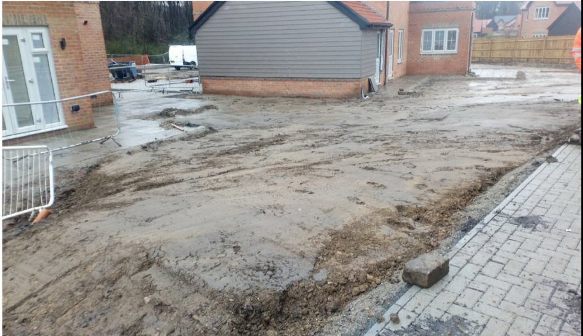
Placement of subsoil on membrane for Plot 174
