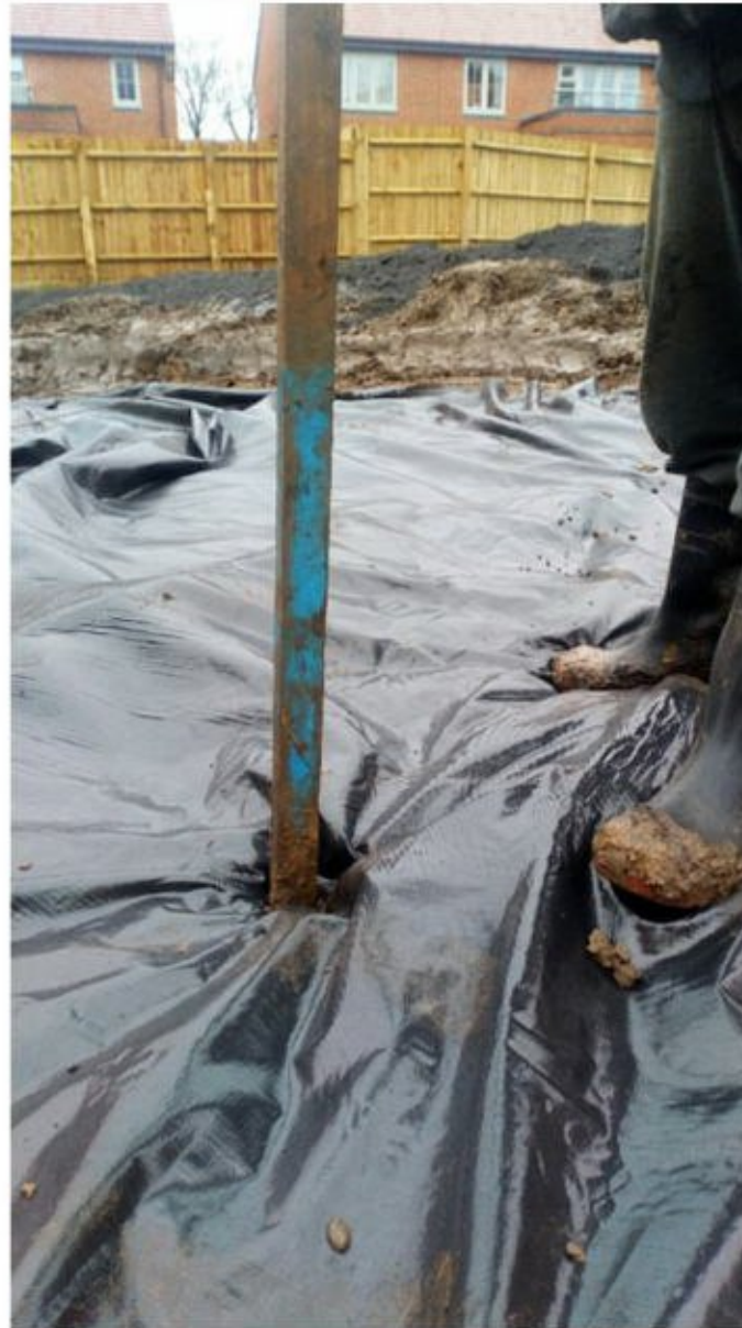
Placement of membrane and measuring 600mm for Plot 174
