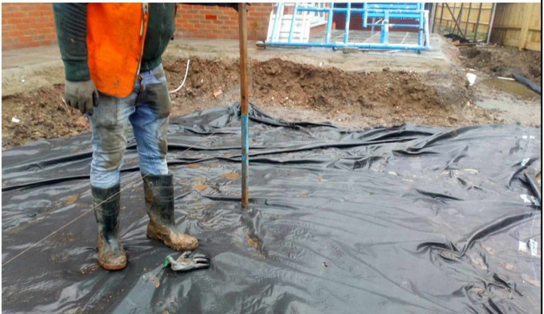
Correct depth being measured for subsoil on plots
