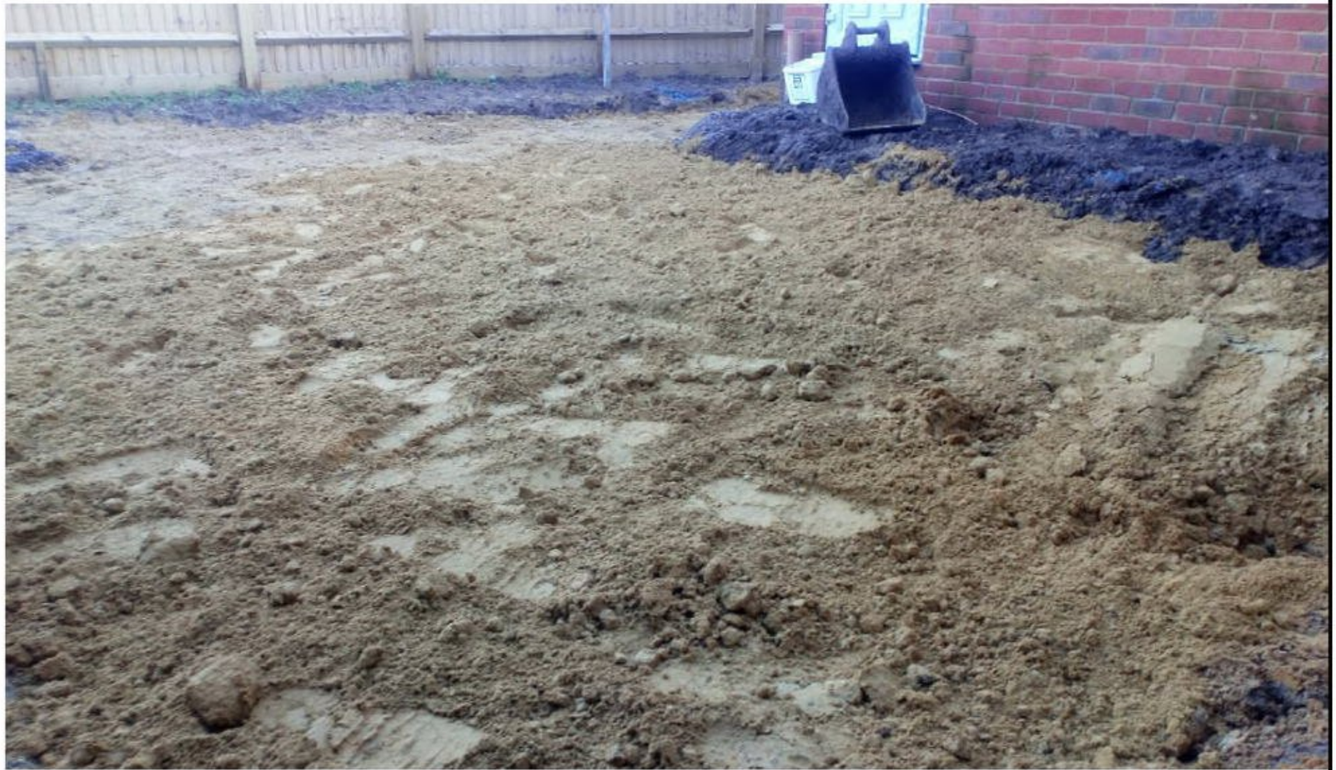
Subsoil completed in Plot 177
