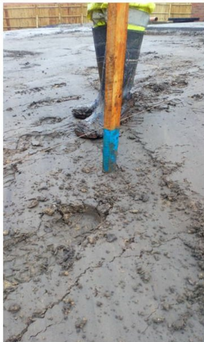
450mm of subsoil placed across Plot 174
