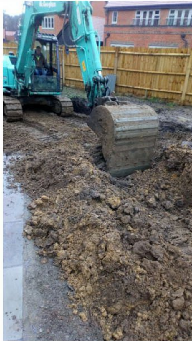
Placement of subsoil on membrane for plots 175 and 176
