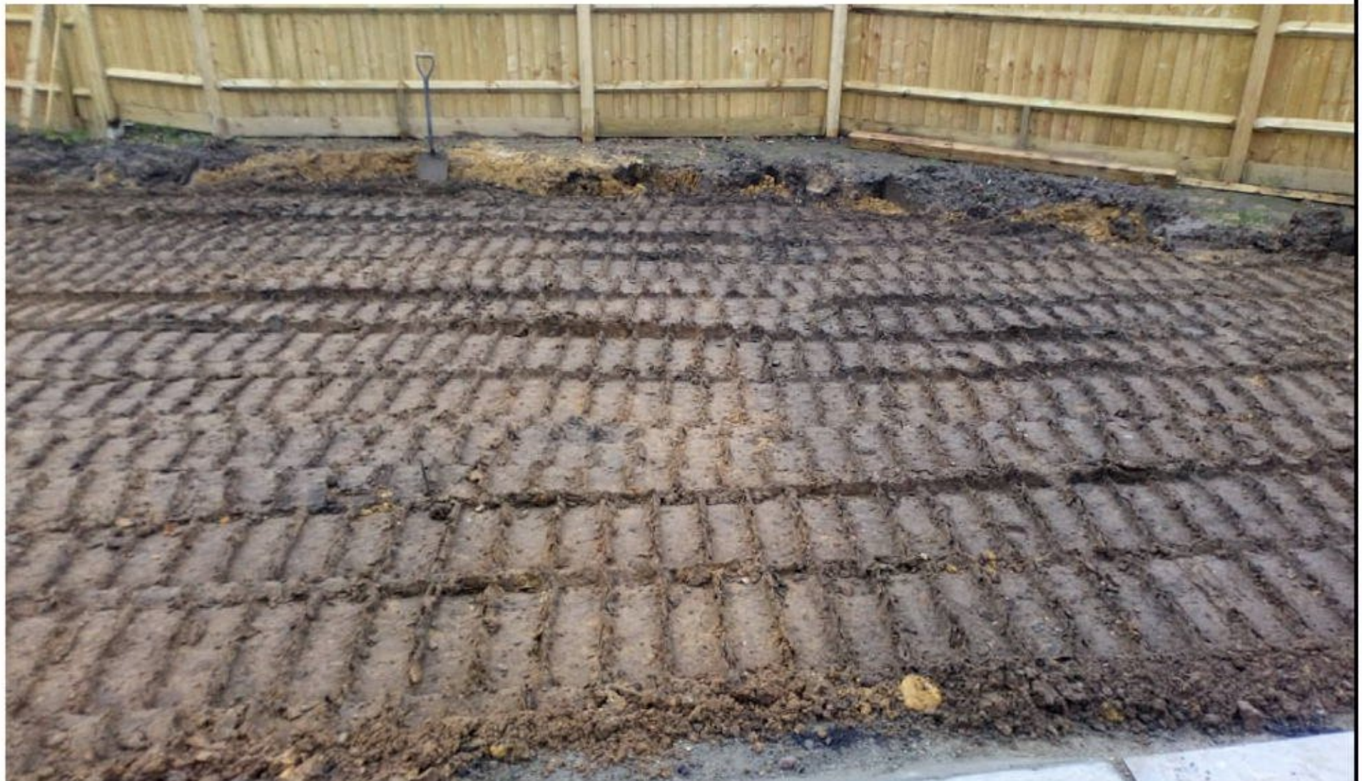
450mm of subsoil placed across Plots 172 and 173
