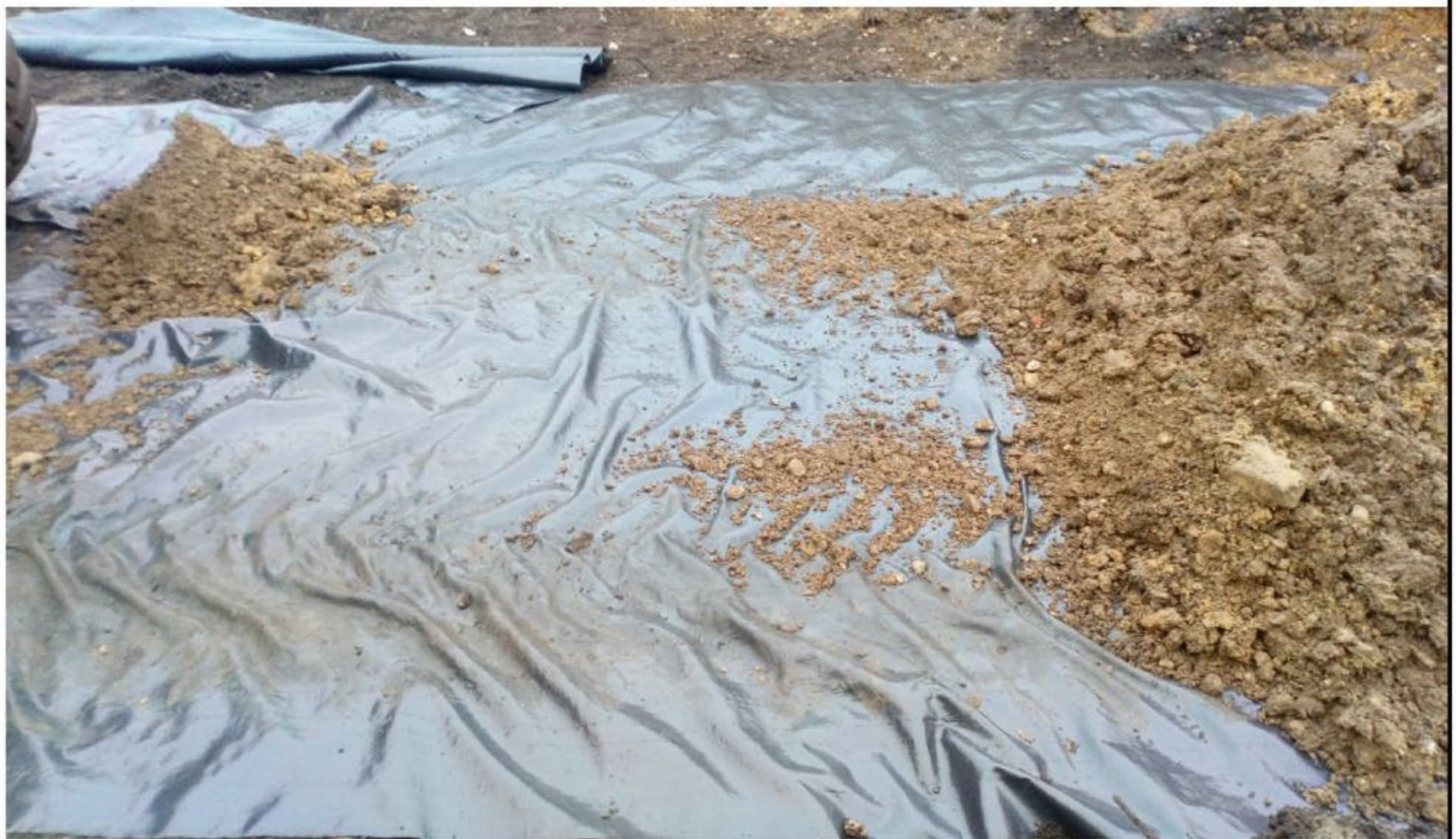
Placement of subsoil on membrane
