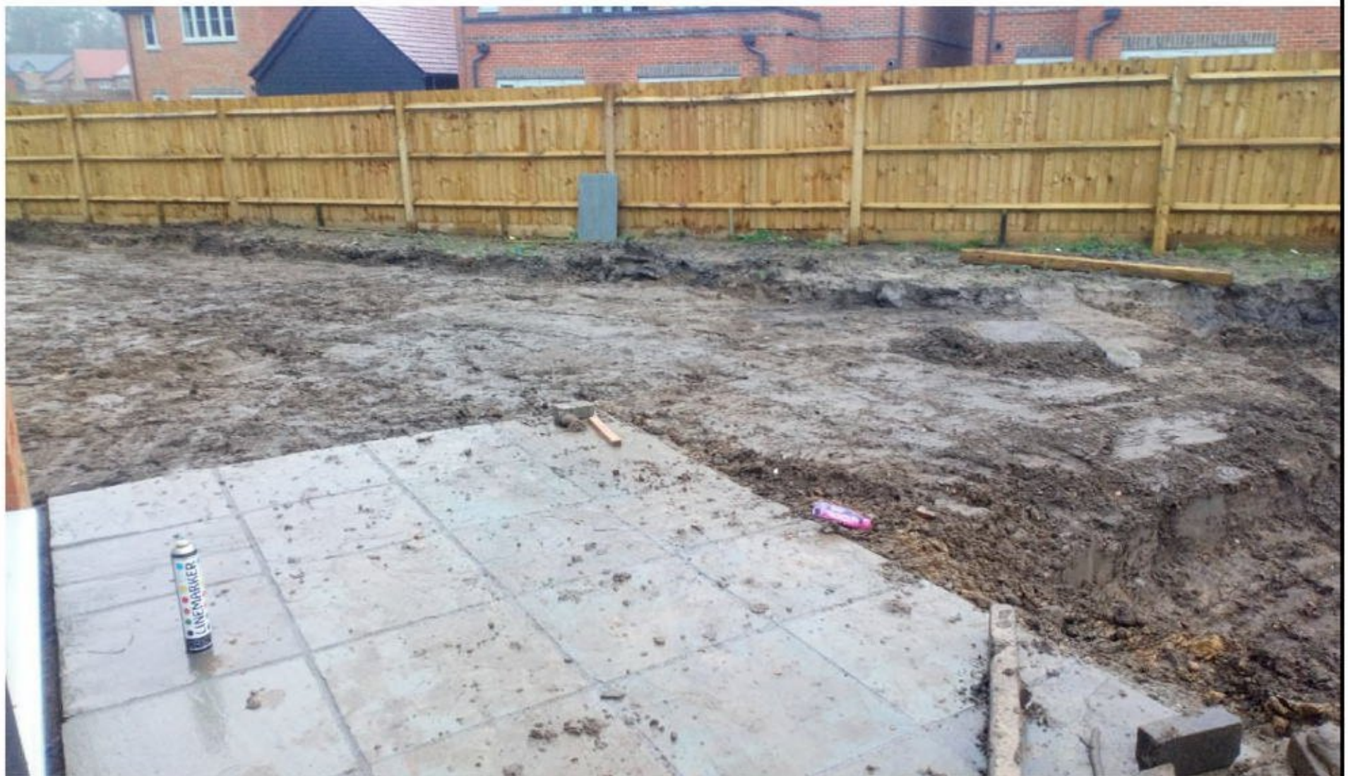
450mm of subsoil placed across Plots 175 and 176
