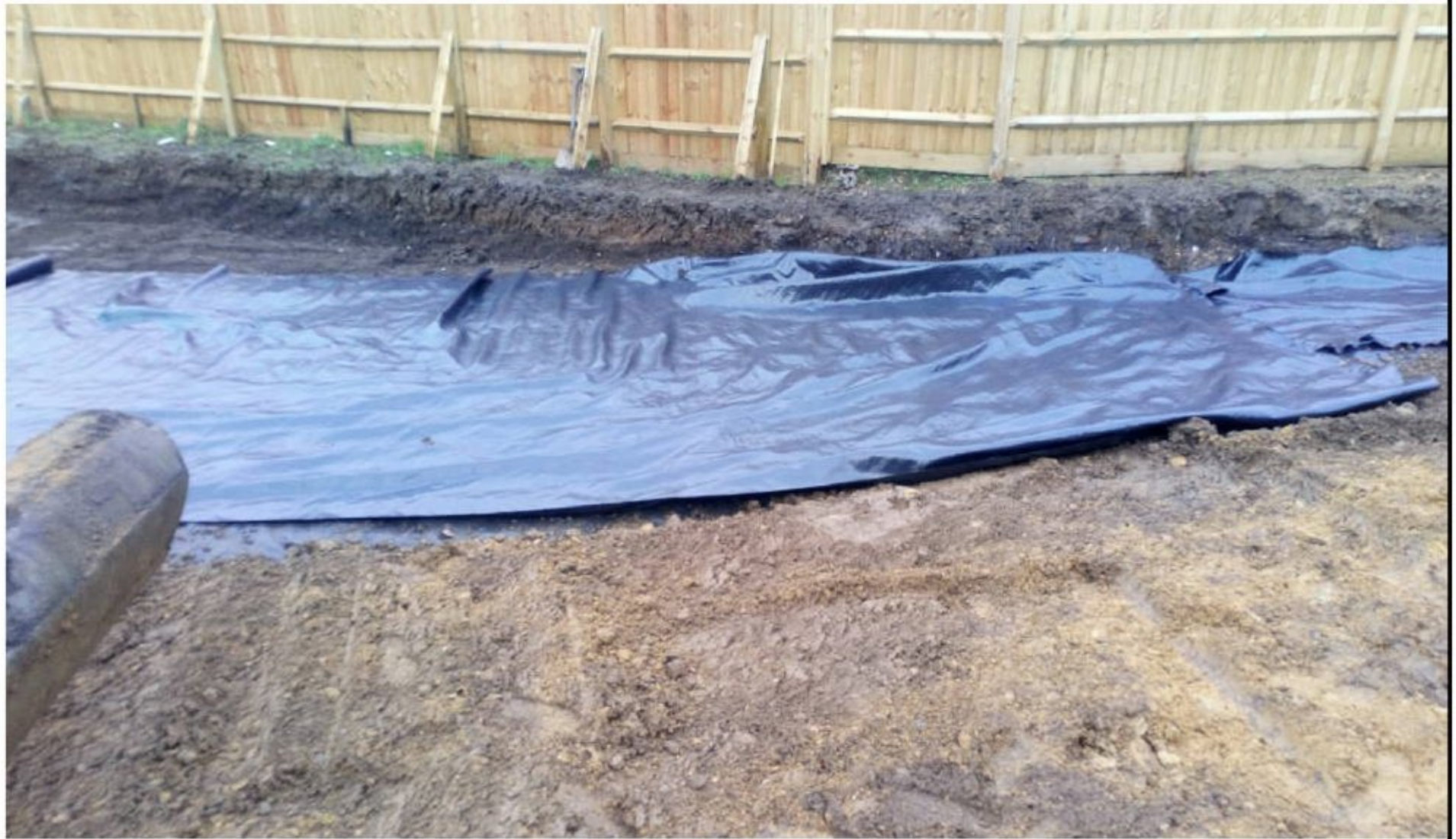
Placement of membrane in Plots 172 and 173
