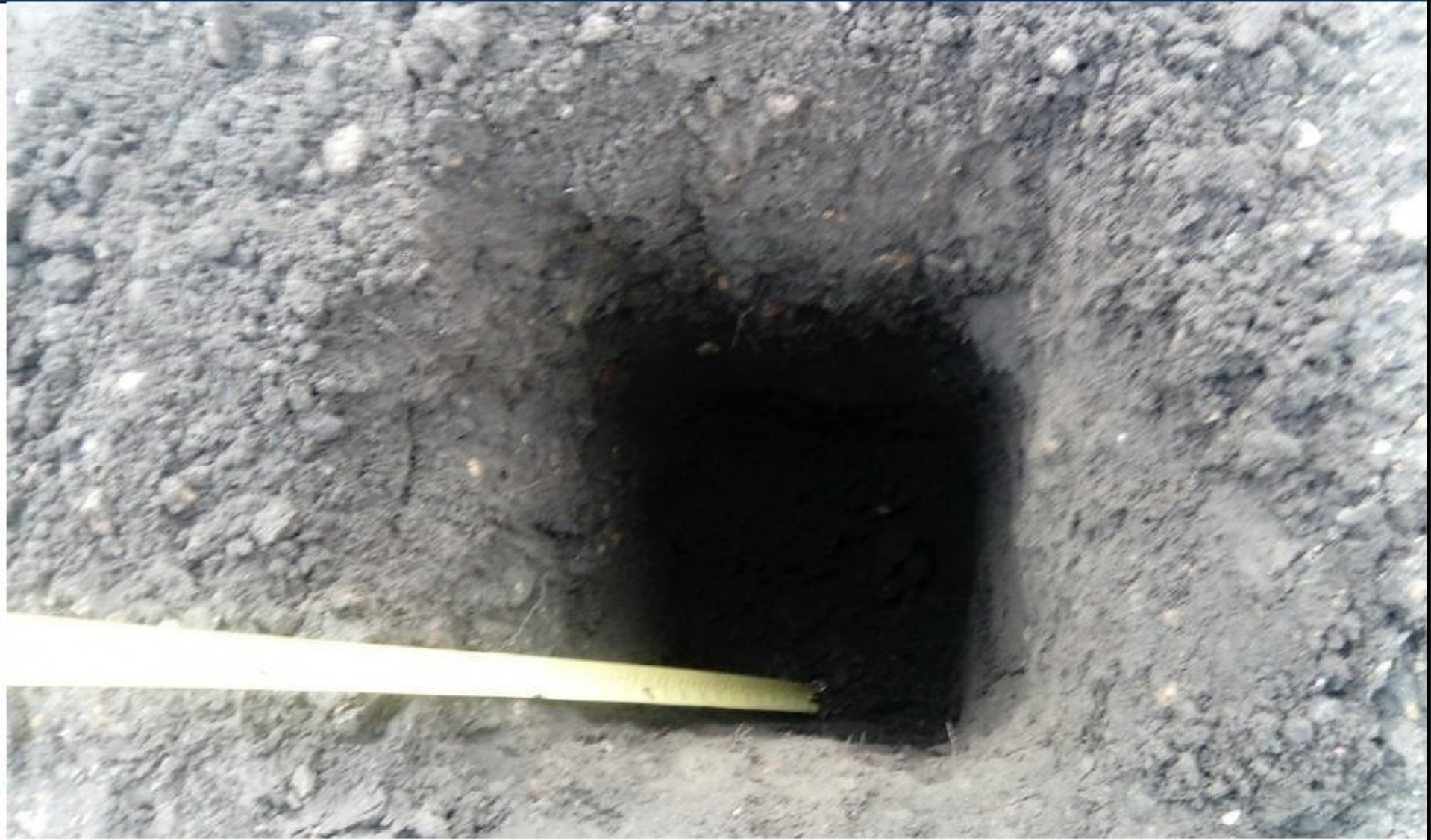
Plot 27A hand excavated pit
