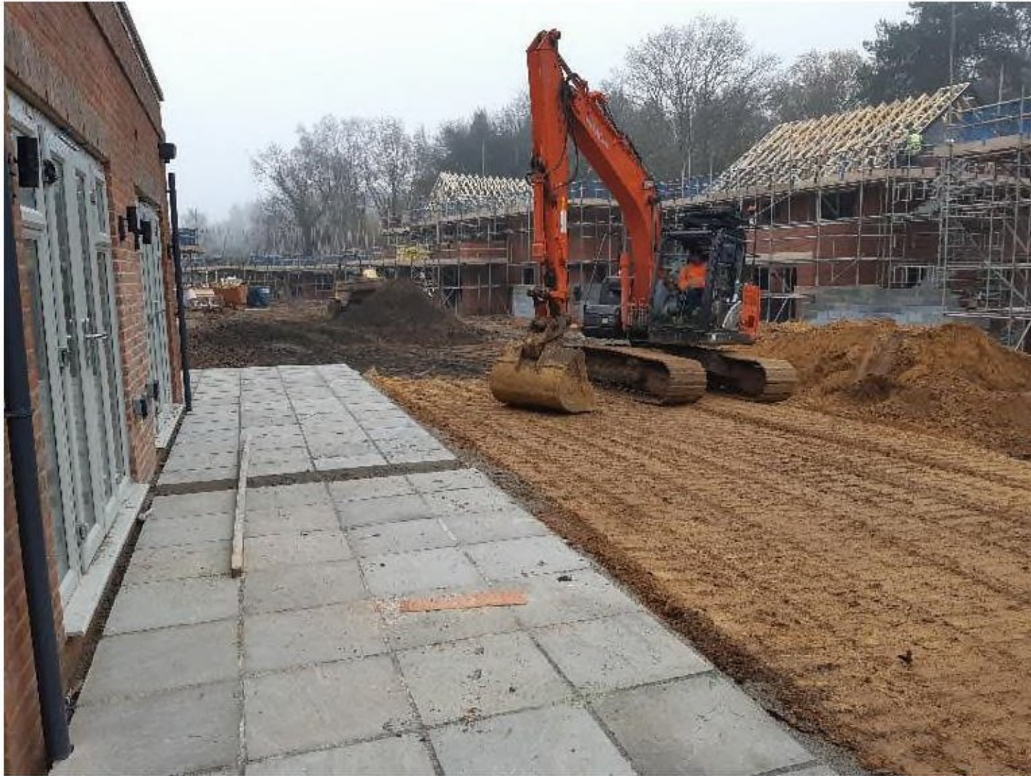
Tracking placed topsoil in Plot 184 + 185.
