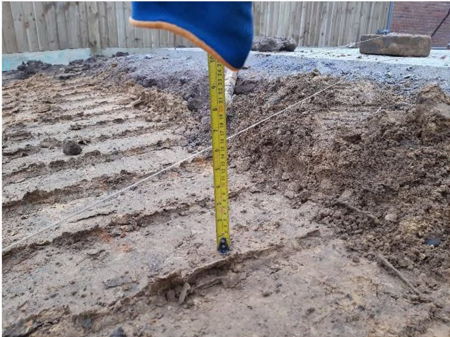
Space left for topsoil in Plots 184 + 185.
