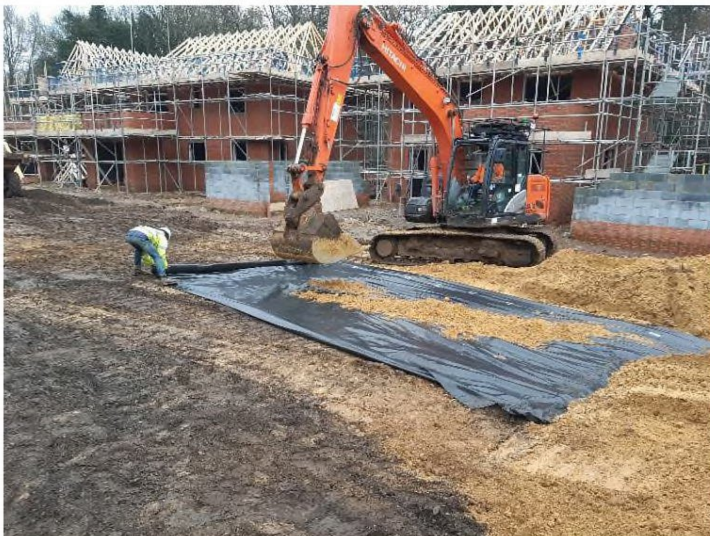
Membrane being laid for Plots 186 (right) and 187 (left).
