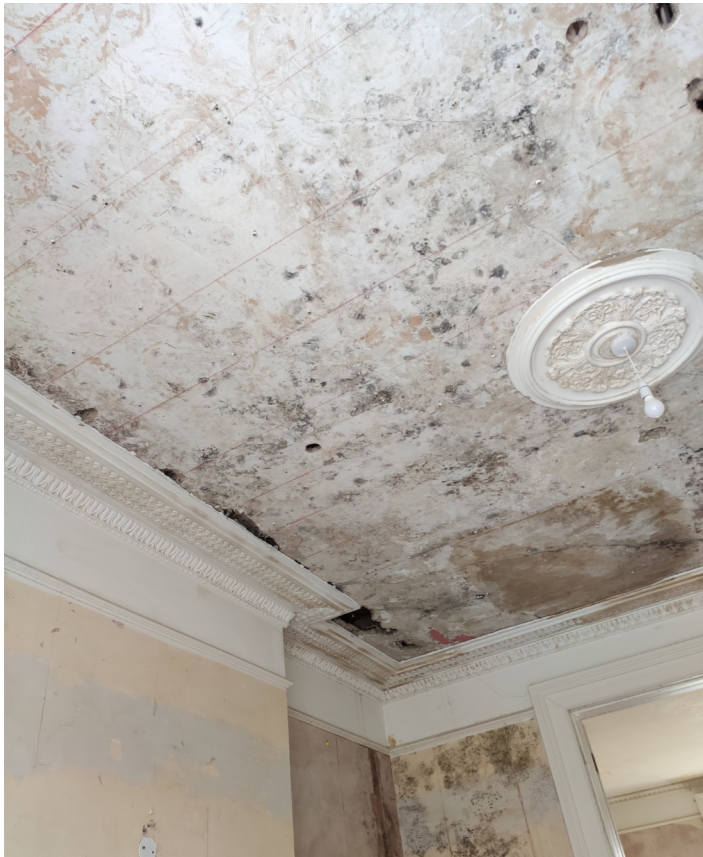
FIGURES 4 - DINING ROOM EXISTING LATH AND PLASTER CONDITION - WATER DAMAGED AREAS OF CEILING TO BE REPLACED. EXISTING HOLES IN PLASTER TO BE REPAIRED, PLASTER TO BE REINSTATED.
