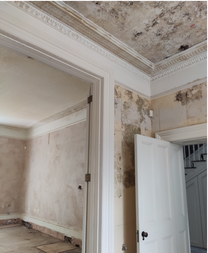
FIGURES 7 - DINING ROOM EXISTING LATH AND PLASTER CONDITION - WATER DAMAGED AREAS OF CEILING TO BE REPLACED. EXISTING HOLES IN PLASTER TO BE REPAIRED, PLASTER TO BE REINSTATED.
