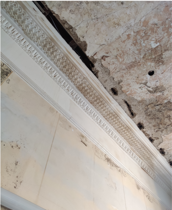
FIGURES 6 - DINING ROOM EXISTING LATH AND PLASTER CONDITION - AREAS OF MISSING PLASTER TO BE REINSTATED. CRACKS IN PLASTER TO BE REPAIRED.
