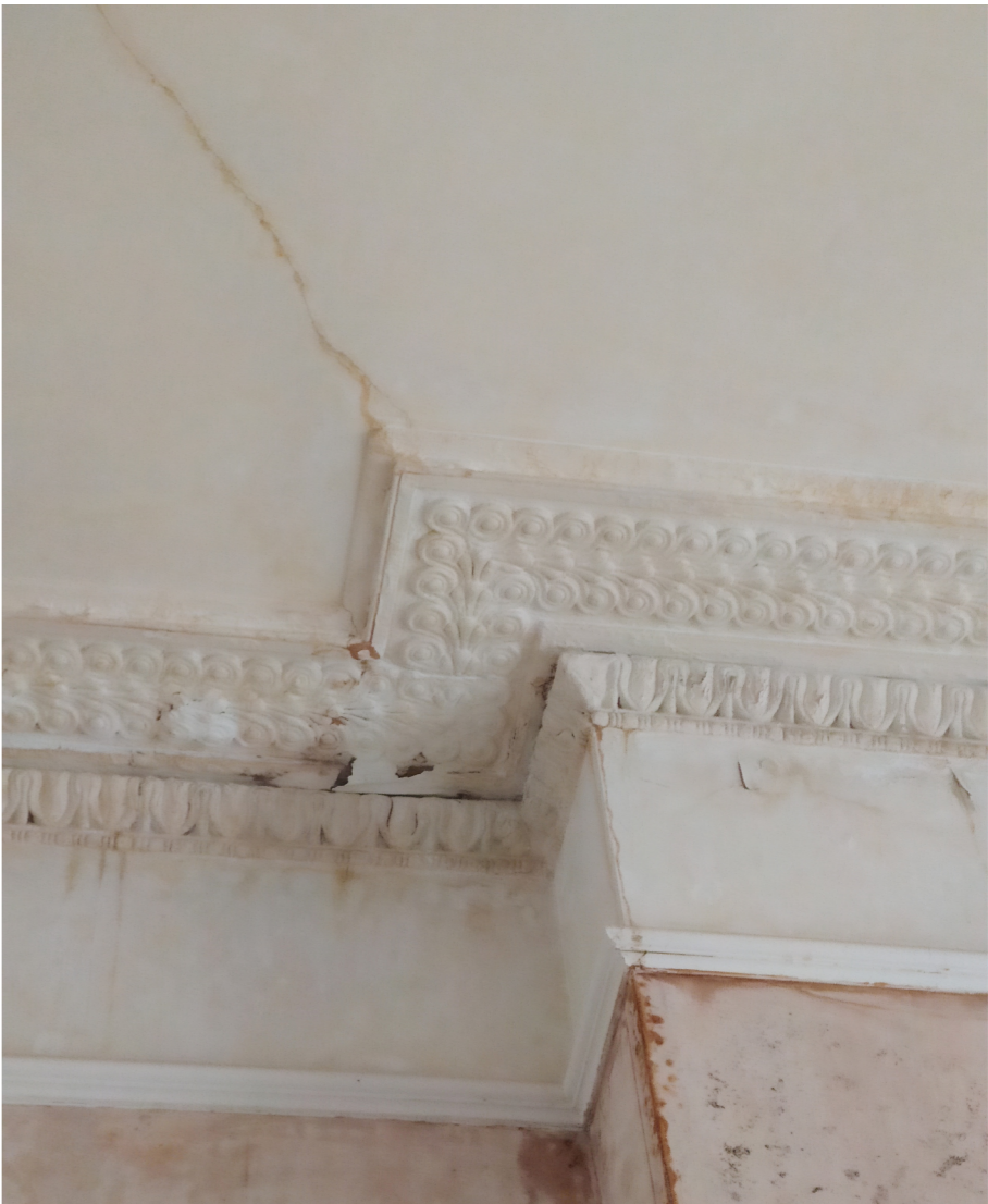
FIGURE 3 - LIBRARY EXISTING CONDITION - CRACKS IN PLASTER TO BE REPAIRED. WATER DAMAGED AREAS TO BE REPLACED.
