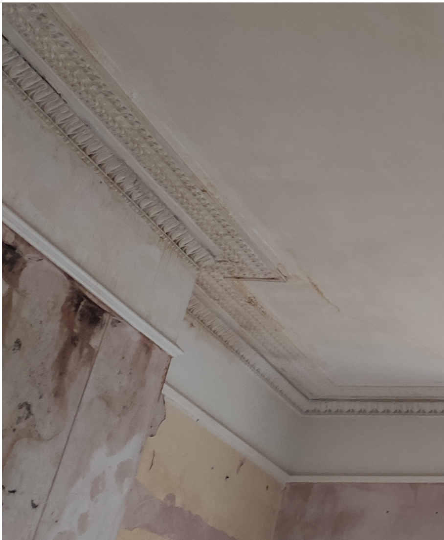
FIGURE 1 - LIBRARY EXISTING CONDITION - WATER DAMAGED AREAS OF CEILING BY THE CORNICE TO BE REPLACED.
