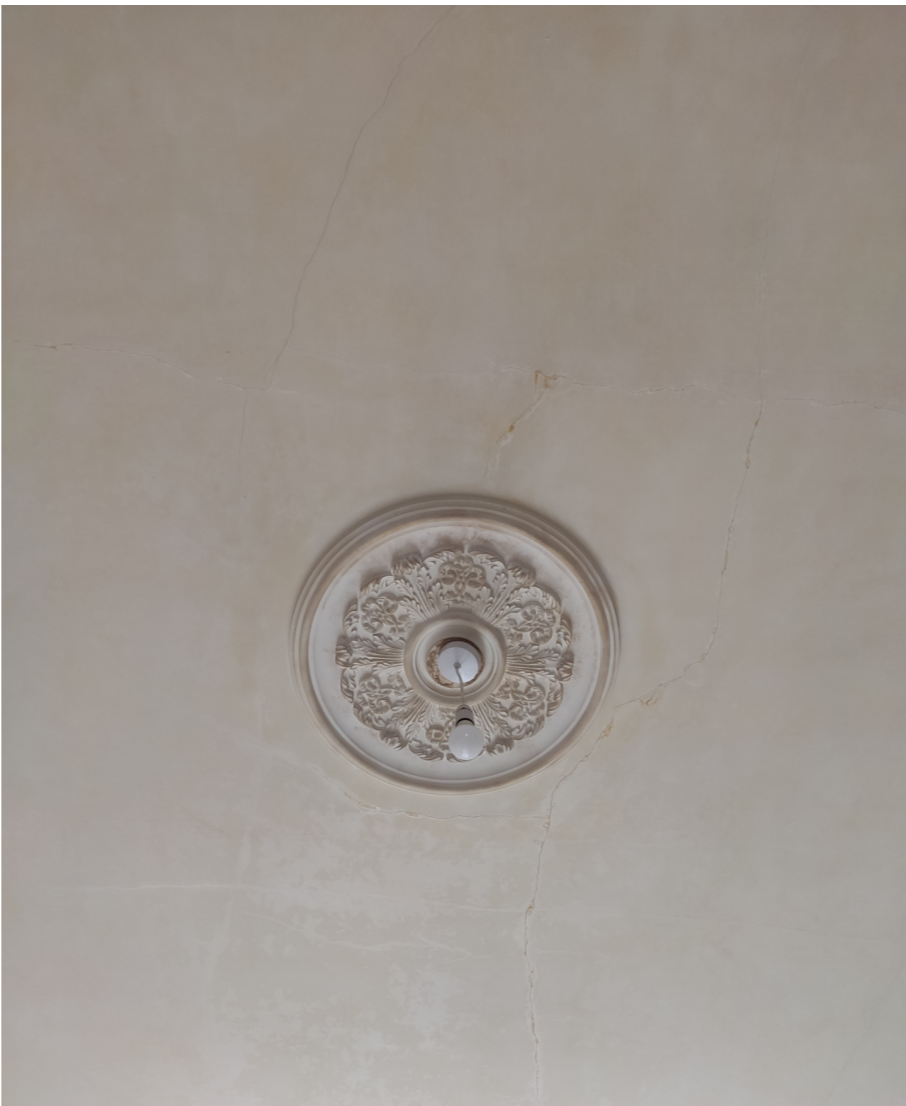
FIGURE 2 - LIBRARY EXISTING CONDITION - CRACKS IN PLASTER TO BE REPAIRED.
