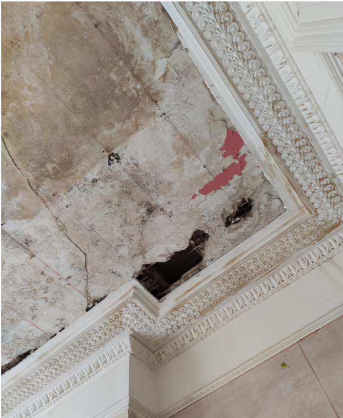
FIGURES 5 - DINING ROOM EXISTING LATH AND PLASTER CONDITION - AREAS OF MISSING PLASTER TO BE REINSTATED. CRACKS IN PLASTER TO BE REPAIRED.
