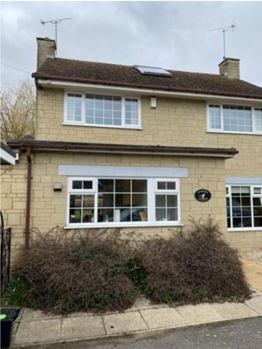
Photograph 2 – View looking north-west showing current window which is to be infilled to create the new front door position with a lean-to roof over.
