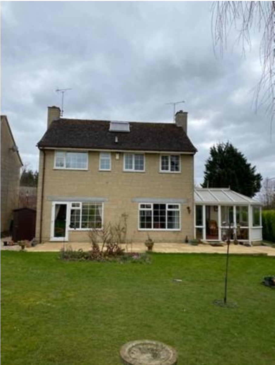
Photograph 4 – View looking south-east showing rear elevation with conservatory to right hand side to be removed this is the position of the proposed two storey extension.
