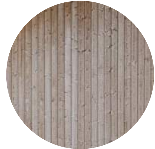
Vertical timber cladding
