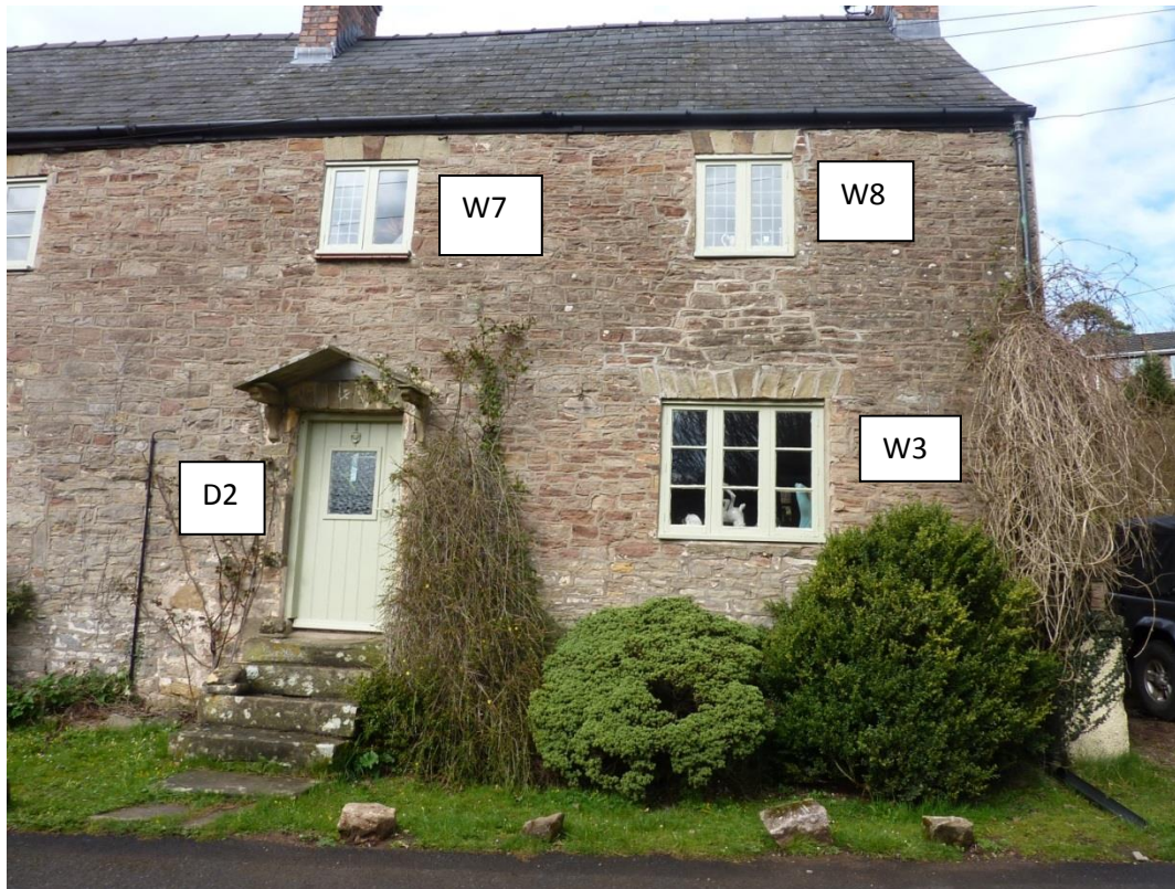
FIG 4: Front south elevation (Vine Tree Cottage)
