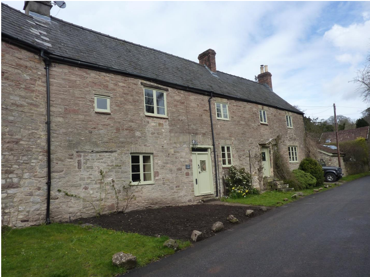
FIG 1: Front South elevation; Laundry Lane
