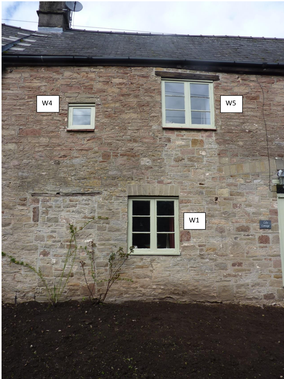
FIG 7: W1 (Ground floor). W 4 & W5 (First floor)
