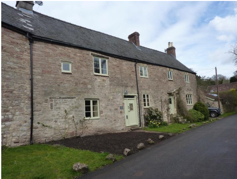
FIG 1: Front South elevation; Laundry Lane
